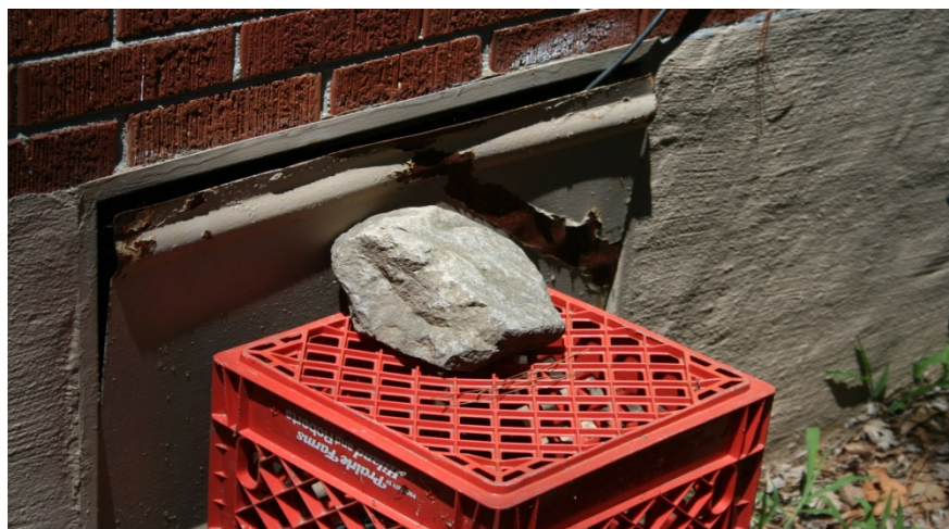
The picture above shows an unsecured and damaged crawl space door.
