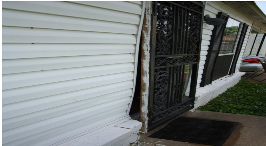
The picture above shows an exterior storm door frame pulling away from the exterior of the unit.
