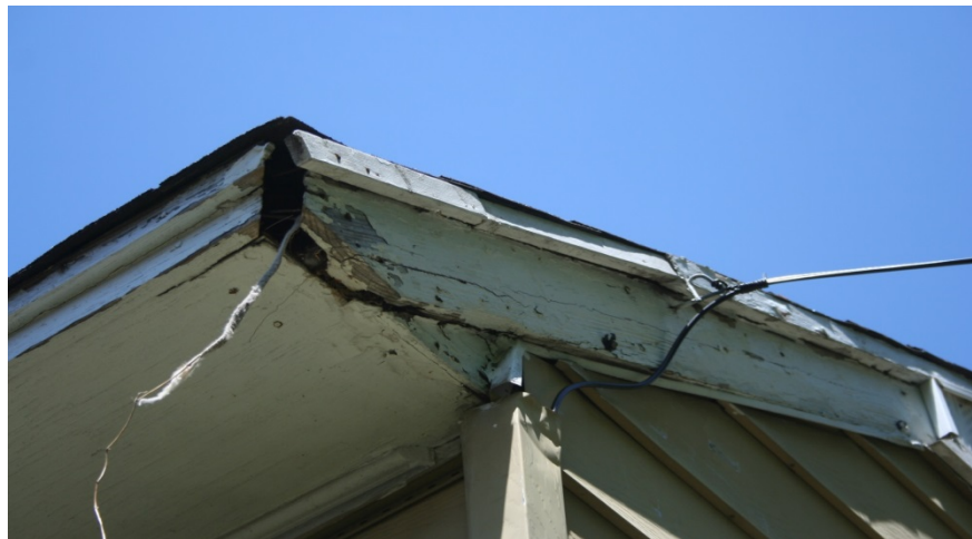
The picture above shows rotted and deteriorated fascia.
