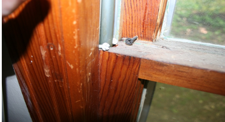
The picture above shows a bedroom window screwed shut, blocking egress from room in the event of emergency, such as fire.
