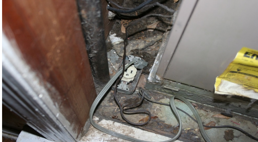
The picture above shows exposed wiring on an inappropriately installed electrical outlet.
