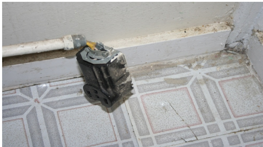
The picture above shows an incorrectly installed high-voltage outlet, which is hanging from its electrical wiring.
