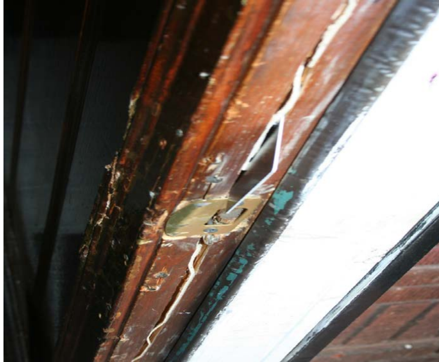
The picture above shows an entry door frame severely damaged, not allowing for adequate unit security.
