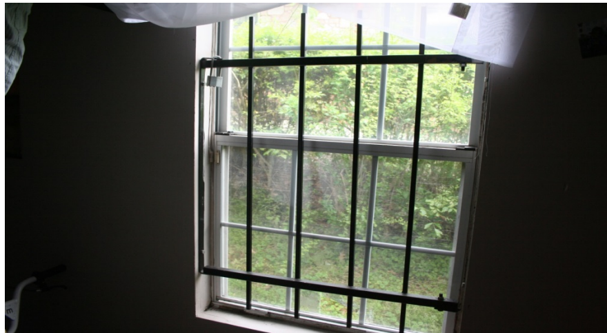
The picture above shows iron bars on the bedroom window, which is locked with a keyed padlock, potentially blocking egress in case of emergency, including fire.
