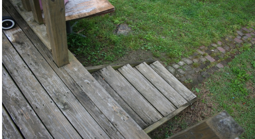
The picture above shows a missing exterior handrail on exterior steps.
