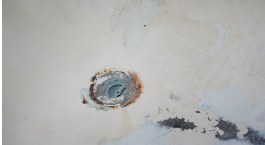
The picture above shows a damaged and rusted tub drain with peeling and chipped tub finish
