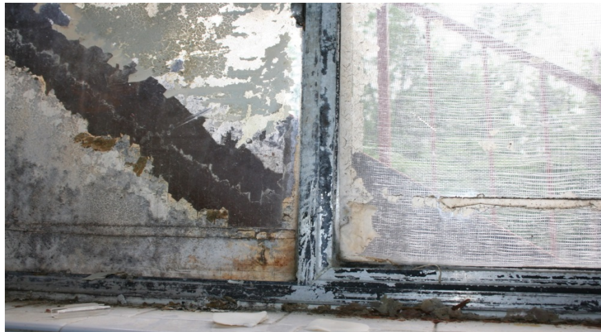
The picture above shows a severely deteriorated bathroom window frame, including peeling paint and mold and mildew buildup.
