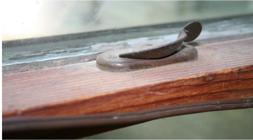
The picture above shows a broken first floor window lock (missing piece of lock on window frame).
