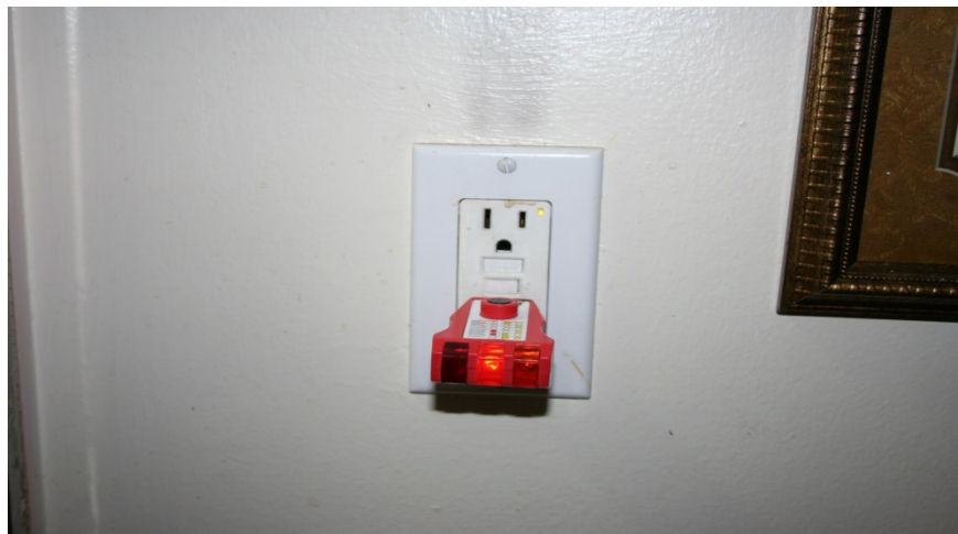
The picture above shows an incorrectly wired ground fault circuit interrupter.
