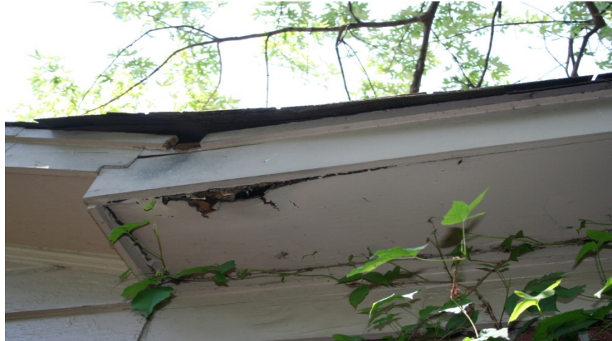
The picture above shows rotted fascia and soffit.
