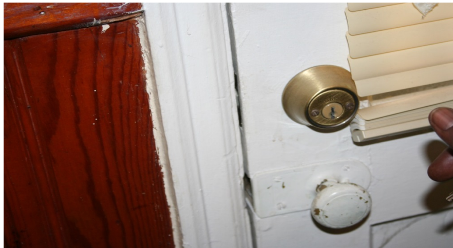
The picture above shows a keyed dead-bolt lock on an exterior door. If the tenant cannot find the key, egress is blocked in case of emergency, such as fire.
