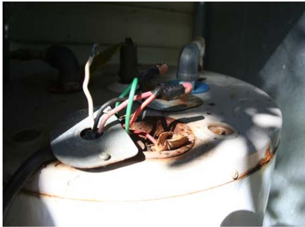
Inspection #11: Top and sides of the hot water heater were corroded due to improper installation.
