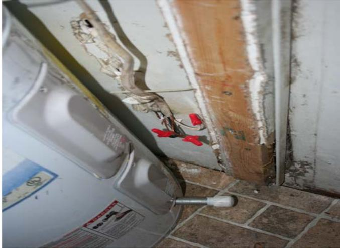
Inspection #4: Heating and electrical systems had exposed electrical wiring.
