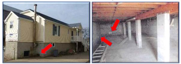
Figures 3 and 4: Subject property exterior and interior pictures showing wash-out floor flood vents (see red arrows)
