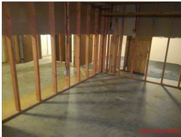
Photo showing that drywall has been removed.
