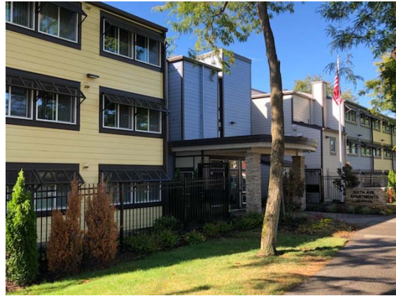
Figure 2 Sixth Avenue Apartments
