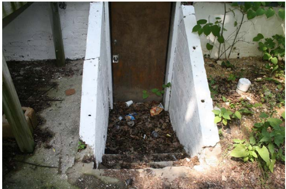
Unit 46: Stairs to basement; no handrail, stairs covered in debris, and dangerous tripping hazard
