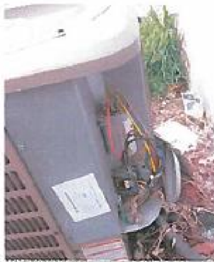
Exhibit 19: 911 Longworth St Open AC compressor compartment 166 days after NHA inspection
