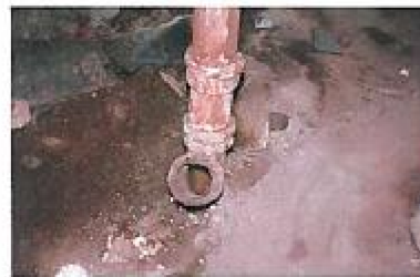
Inspection 4: One of two open sewers in the basement, creating a health hazard because of harmful sewer gases escaping. The Authority did not identify this violation during its December 13, 2017, inspection.
