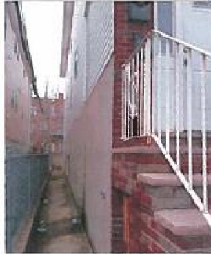
Exhibit 21: Unit 12 Missing downspout section 166 days after NHA inspection
