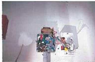
Inspection 24: An open junction box in the first floor stairwells creates a risk of electrical shock and injury. The Authority did not identify this violation during its October 10, 2017, inspection.
