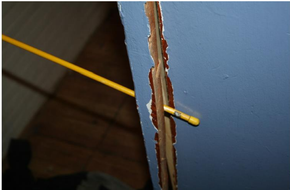
Inspection 29: A cracked rear entry door jamb, posing a threat to space and security. The Authority did not identify this violation during its November 2, 2017, inspection.
