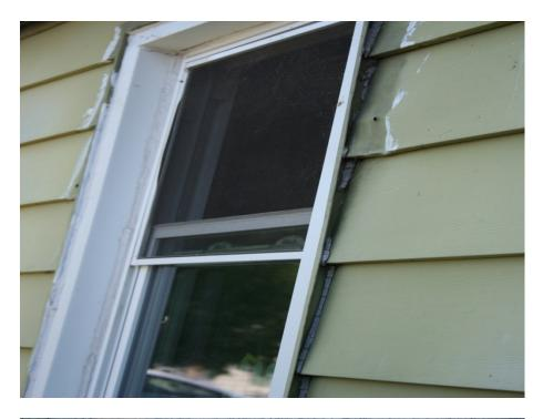
Project number 3704: Window sash not repaired or completely painted
