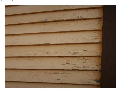
Project number 3692: Existing paint not properly scraped, paint applied over existing peeling paint, and paint peeling
