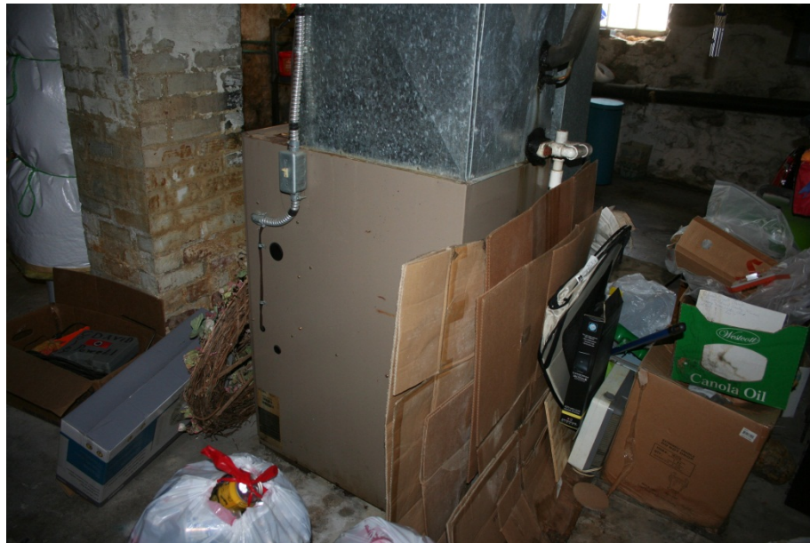
Unit #6: Household personal items stored around gas heating equipment
