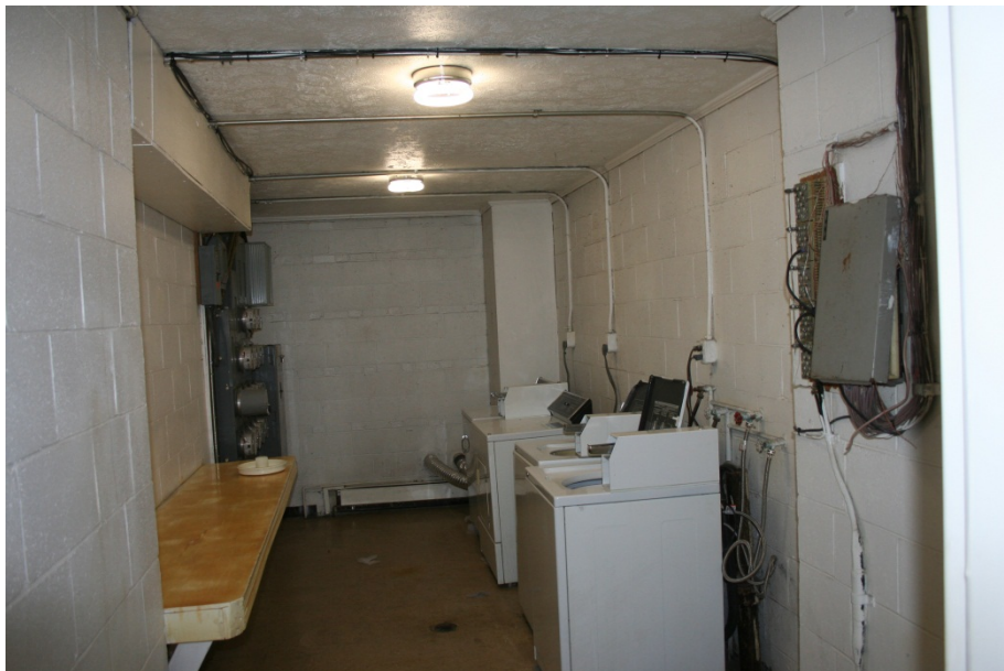
Unit #42: Exposed high tension electrical wiring, reachable to tenants and children, in building laundry room facility
