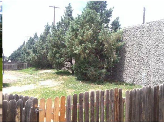
Sound wall in back of townhomes
