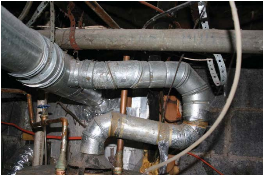
Inspection #32: The vent on the hot water heater had a negative slope, which prohibited gases from venting properly. The Authority did not identify this violation during its November 5, 2012, inspection.
