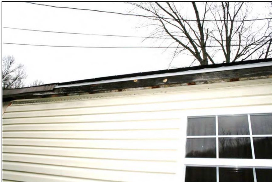
Inspection #76: The soffit on the unit's exterior was missing. The Authority did not identify this violation during its November 8, 2012, inspection.
