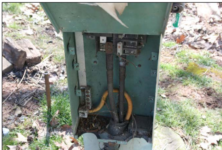
Inspection #16: The breaker box on the unit's exterior was not secure and had exposed electrical contacts with high voltage. The Authority did not identify this violation during its November 26, 2012, inspection.
