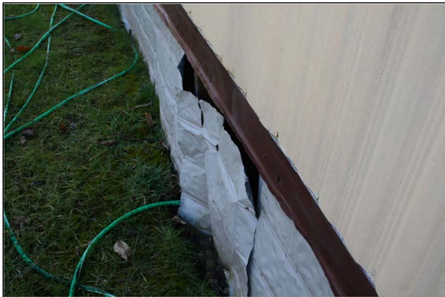
Inspection #21: The skirting on the mobile home exterior was loose and had sharp edges. The Authority did not identify this violation during its November 9, 2012, inspection.
