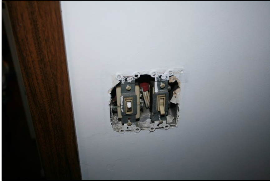
Inspection #54: The electrical outlet in the hallway was missing a cover. The Authority did not identify this violation during its November 8, 2012, inspection.
