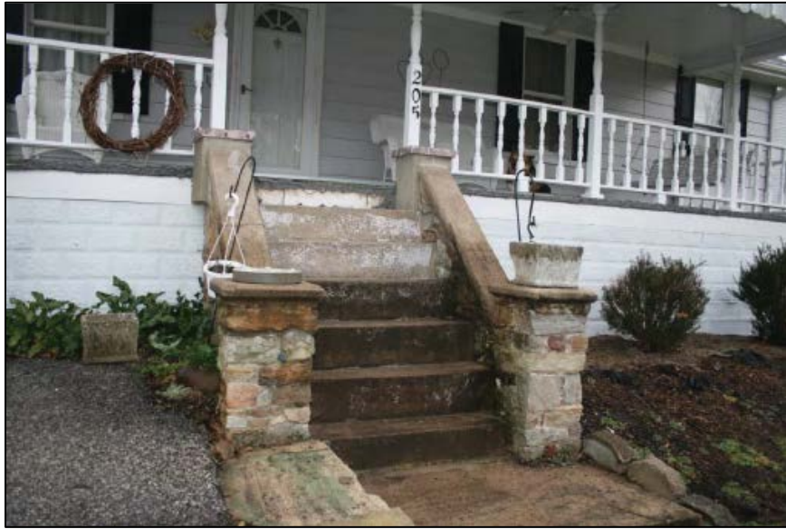
Inspection #20: The exterior staircase was missing a handrail. The Authority did not identify this violation during its November 9, 2012, inspection.
