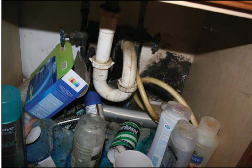
Inspection #22: There was a hole in the wall and possible mold and mildew under the bathroom vanity. The Authority did not identify this violation during its November 9, 2012, inspection.
