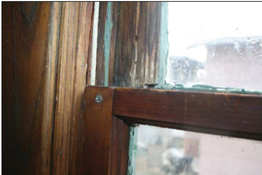
Inspection #40: The window in the bedroom was screwed closed. The Authority did not identify this violation during its November 7, 2012, inspection.
