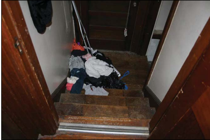
Inspection #32: The stairwell to the basement was missing a handrail. The Authority did not identify this violation during its November 5, 2012, inspection.
