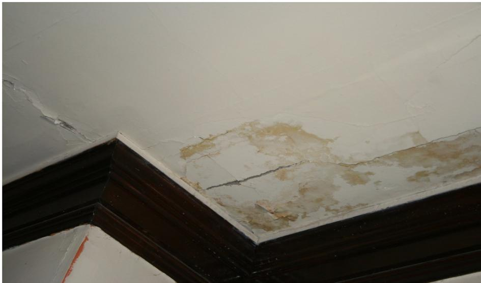
Property number 65 – The roof still leaked after being replaced.
