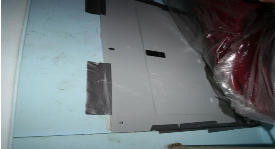
Property number 50 – The electrical service panel was not properly secured by screws to the house studs. The panel was being held in place by duct tape.
