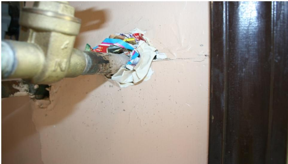
Property number 40 – Drywall was removed to access the water heater; however, after reinstallation of the water heater, the contractor did not repair the damaged exposed wall.
