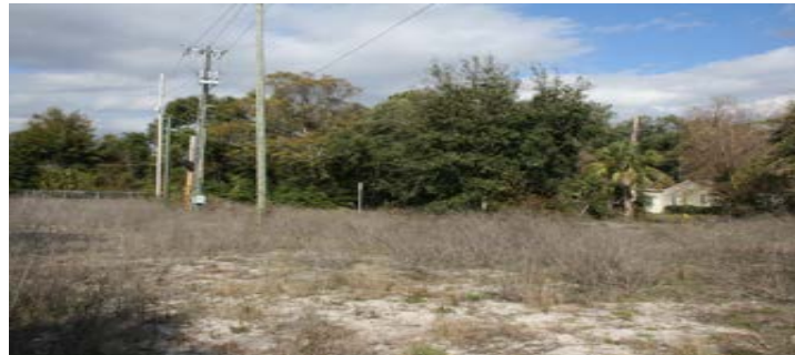
Picture 1: Power lines on project W19
