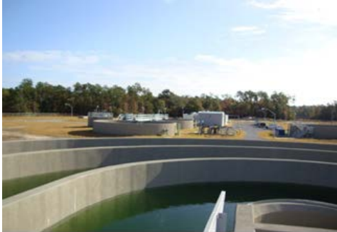
Picture 4: Oxidation Ditch
