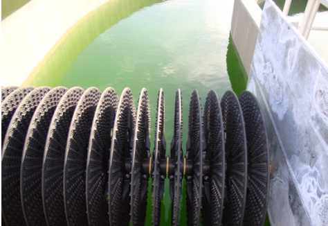
Picture 5: Oxidation Ditch
