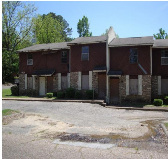
\*\*Property 4 – This property needs Energy Star windows, new hardie board\*\*\* siding, and new roofing shingles.
