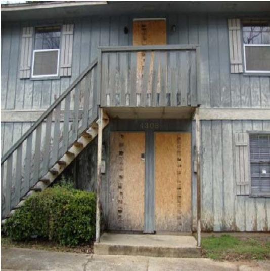
\*\*Property 3– This property needs Energy Star windows and new hardie board siding, and the exterior stairs need to be repaired.
