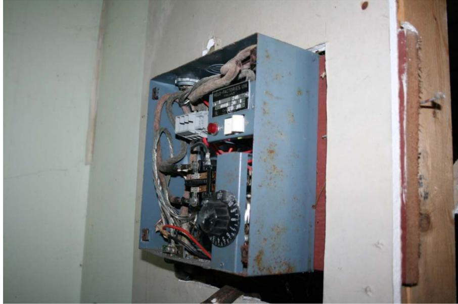
Unit # 8: Electric disconnect box cover not secure, exposing electrical contacts
