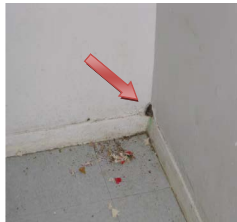
Figure 2: Hole from rodent infestation
