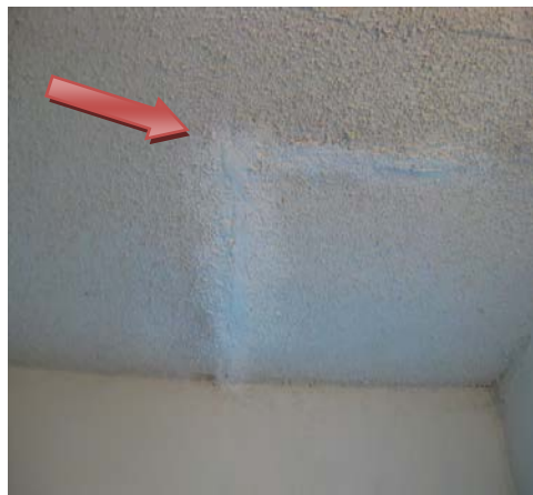
Figure 1: Leaking bathroom ceiling
