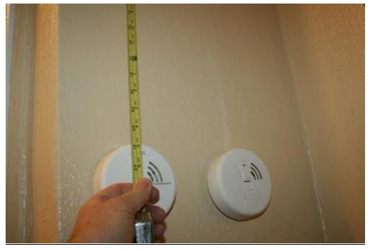
The picture above shows an improperly mounted unit smoke detector. The smoke detector was mounted 41 inches from the ceiling, which was more than the 12-inch requirement, and is considered a possible fire hazard.
