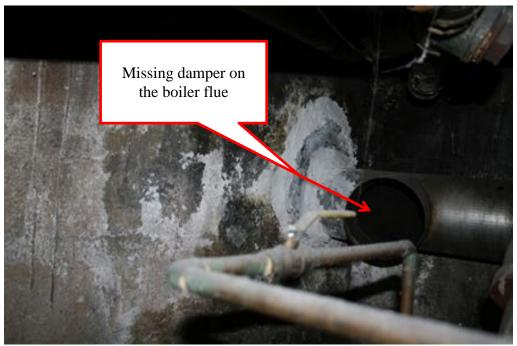
The picture above shows a missing damper on the boiler flue in the basement of a single-family home, which allowed carbon monoxide to reenter the house.
