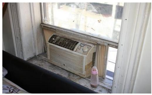
The picture above shows an air conditioning unit not properly secured to the window, which posed a potential falling hazard. Also, there was an open space between the air conditioning unit and the window frame, which presented a falling hazard for a child under the age of 6.
