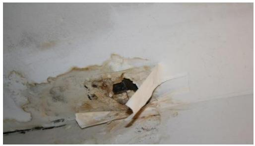
The picture above shows a hole in the unit ceiling above the bathtub. According to the tenant, the hole was patched up by the landlord but continued to leak at times.
