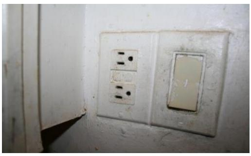
The picture above shows a ground fault circuit interrupter in the bathroom, which did not trip because it was painted over. This unit contained additional violations, such as a light fixture hanging from the wires and not properly secured to the ceiling; excessive grease on the kitchen stove, walls, and cabinets; overcircuiting of outlets; and a rear window that would not stay up.
