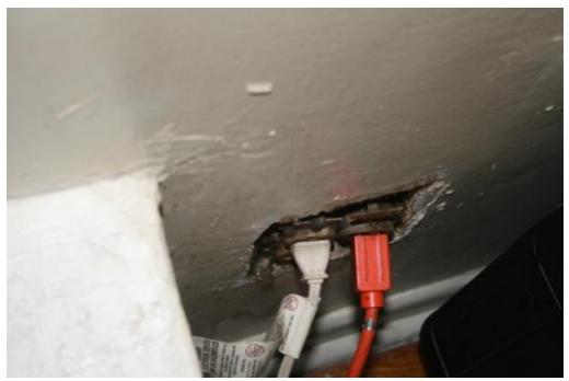
The picture above shows a missing outlet cover in the unit living room. In addition, the outlet was not secured to the junction box.
