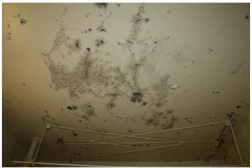
The picture above shows possible mold and mildew stains on the unit bathroom ceiling.
