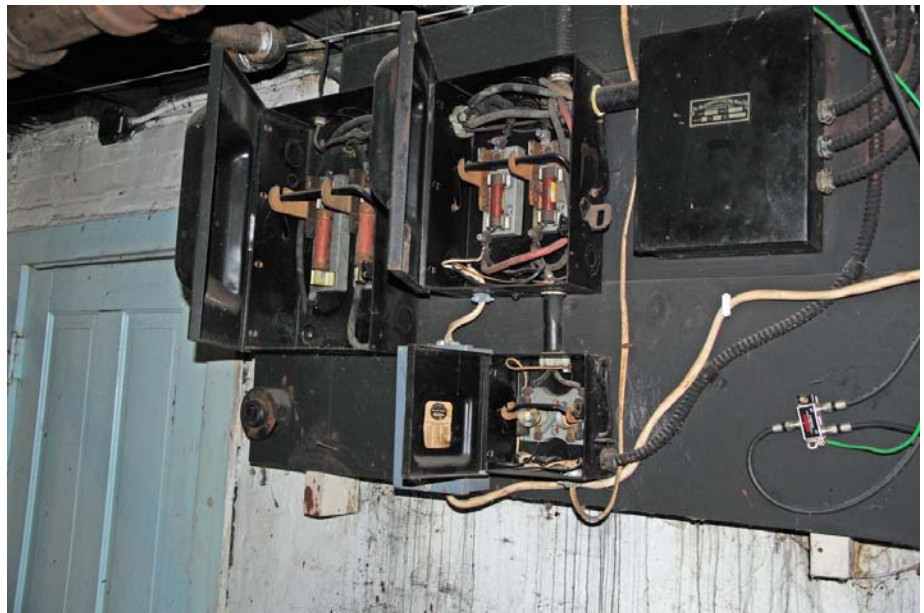
Unit #21: Unsecured power disconnect boxes, exposing electrical contacts
