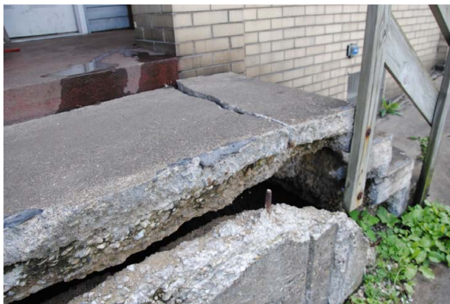
Unit #32: Deteriorated front entrance stoop
