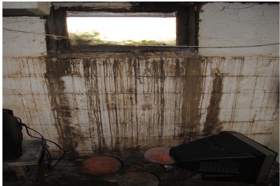
Unit #17: Leaking basement window with the glass pane held in place by duct tape
