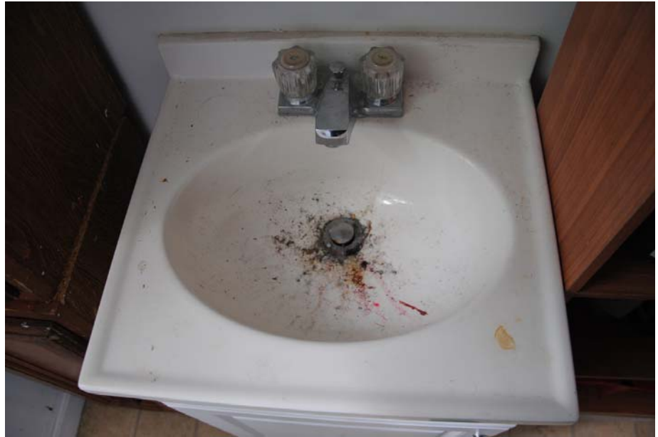
Unit #32: Clogged lavatory drain in only bathroom in house; had not been used since February 2015
