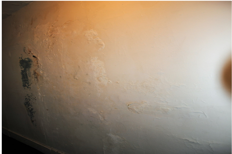
Unit #4: Blisters, cracks, and mold on entry hallway wall
