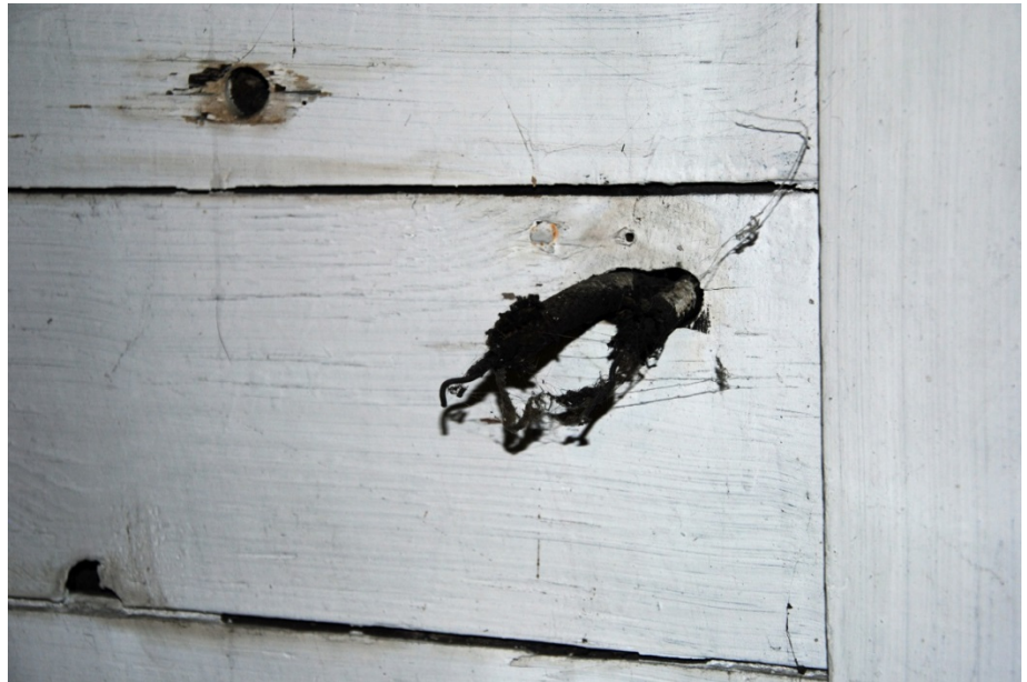
Unit #10: Exposed live wires protruding through a wall
