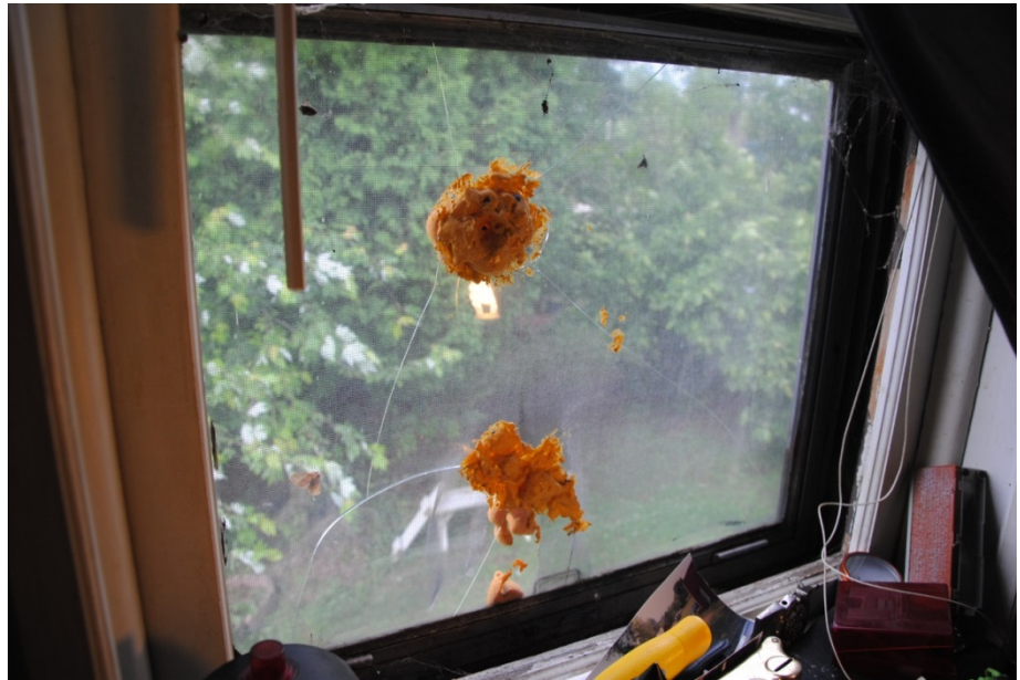
Unit #12: Bedroom window with cracks and holes filled with foam
