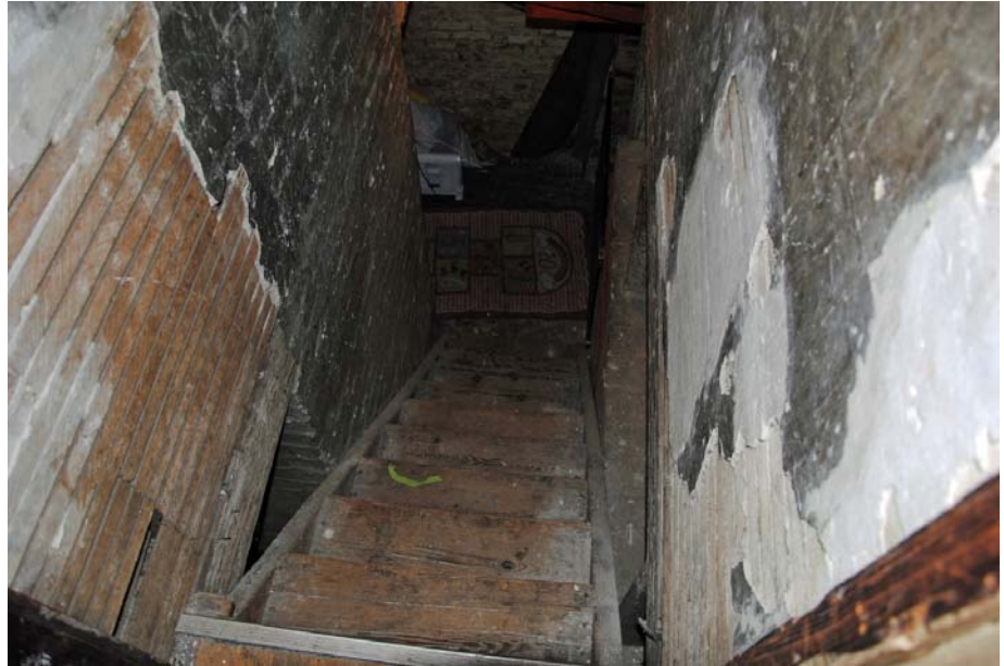
Unit #22: Basement steps with no handrail
