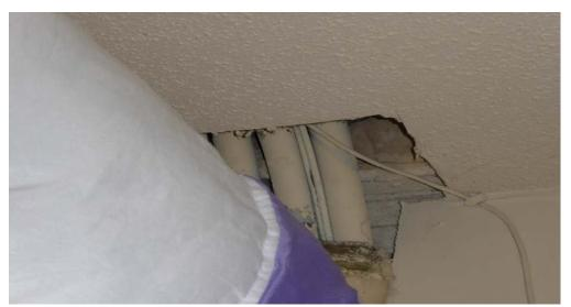
The picture above shows a large hole in a closet ceiling through which pipes are passing. The large hole allows for vermin, dust, and air infiltration.
