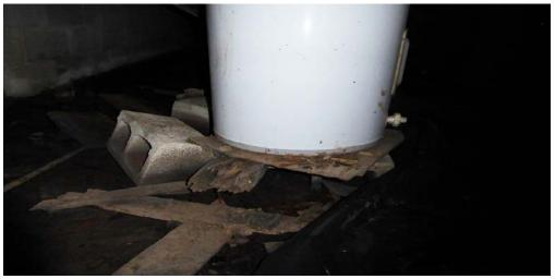
The picture above shows a water heater with an unsteady foundation, allowing it to be easily knocked over, causing injury to tenants or damage to the unit.
