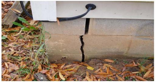
The picture above shows a large crack in the unit's foundation. allowing water, air, and insect infiltration.
