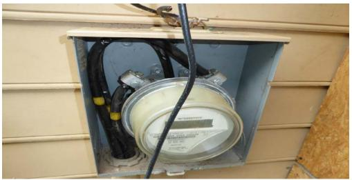
The picture above shows that the cover on an electric meter box is missing the seal and can be easily opened, exposing electrical contacts and creating an electrical hazard such as shock.
