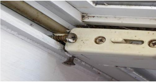
The picture above shows a kitchen window being kept closed with screws, not allowing exit in case of an emergency and not allowing for ventilation.
