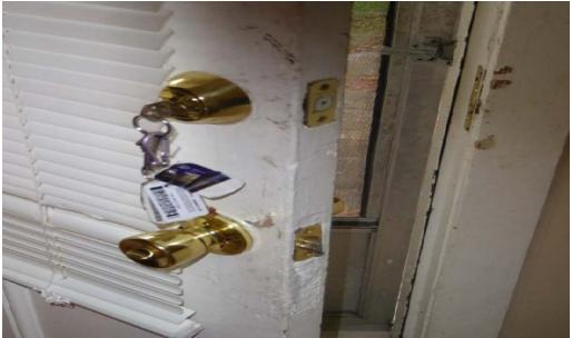
The picture above shows a keyed deadbolt lock on the kitchen exit door. If the tenant cannot find the key, exit would be blocked in case of emergency.
