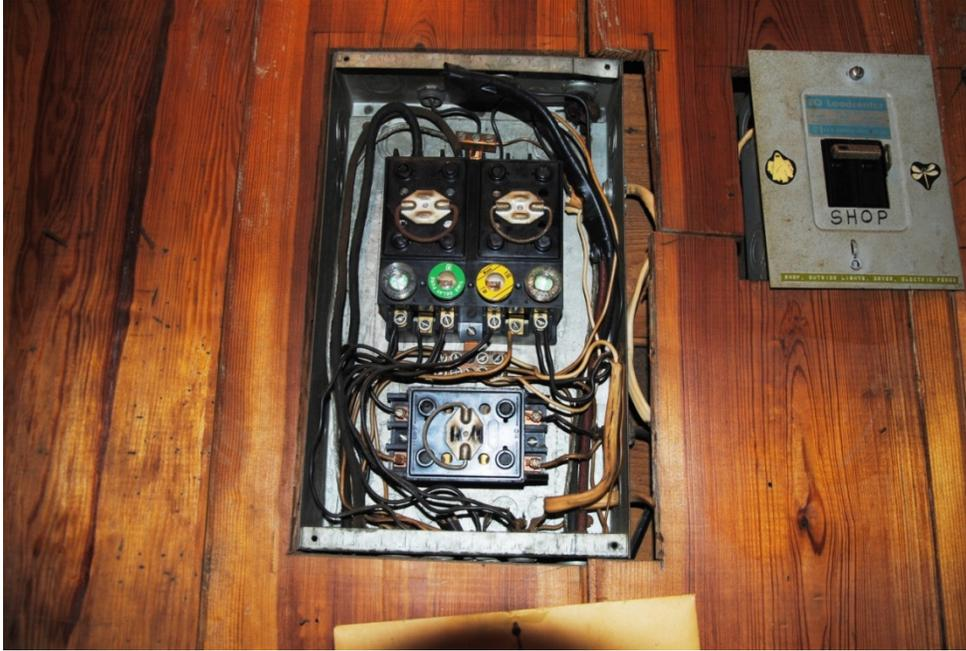
The picture above shows a fuse panel without an internal cover, and the external cover could easily be removed, exposing electrical contacts.
