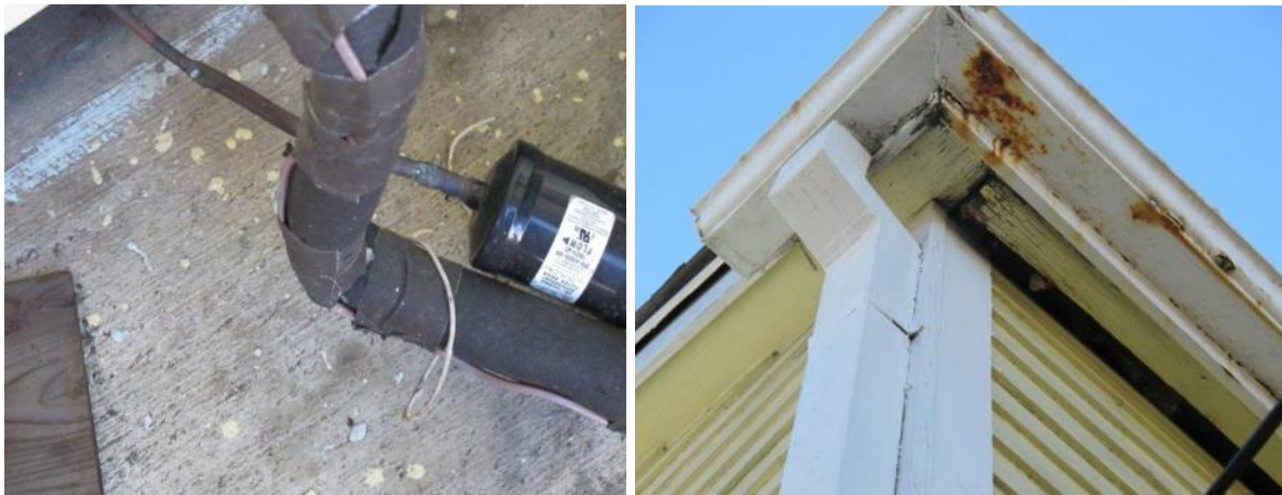
Illustration 2: Exposed wires, damaged gutters, and rotted exterior soffit boards
