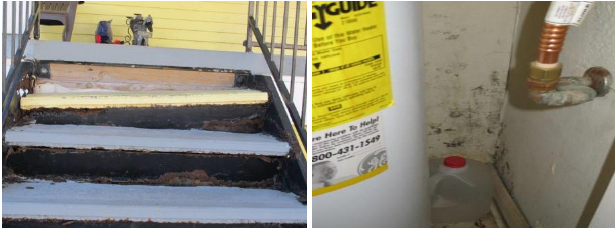
Illustration 1: Rusted staircase with broken step and mold and mildew buildup on walls
