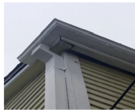
Illustration 2: Repaired of exposed wires, damaged gutter and replaced rotted exterior soffit boards
