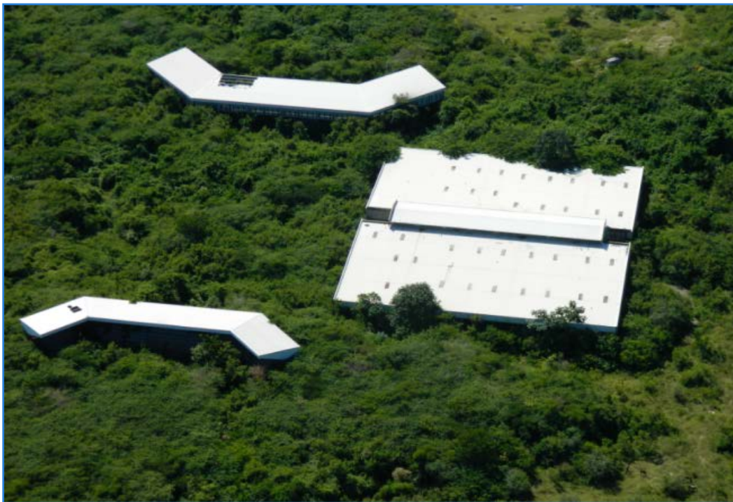
Picture 1 - Audit memorandum 2014-AT-1801, Vieques, PR, a sport complex site was abandoned, and the main recreational building and the baseball facilities were covered with dense vegetation.
