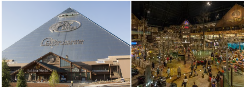
Images of the renovated Pyramid, re-opened as a Bass Pro store in Memphis, Tennessee
