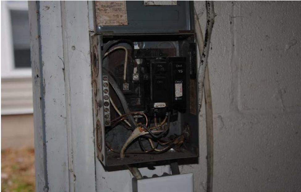
The picture above shows a fuse panel without an internal cover, and the external cover is easily removed, exposing electrical contacts.
