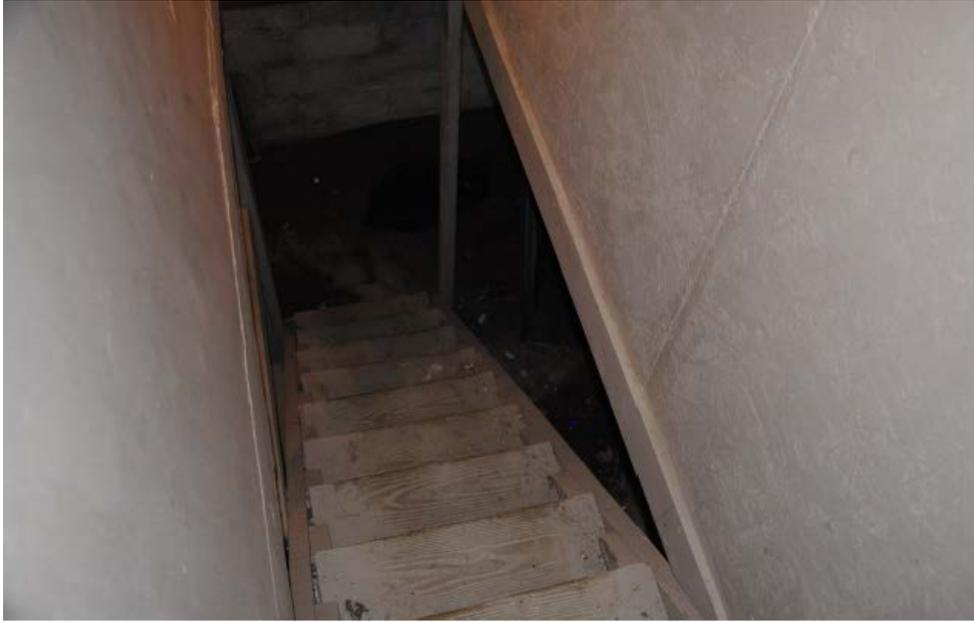
The picture above shows a stairway to the basement that has no handrail.
