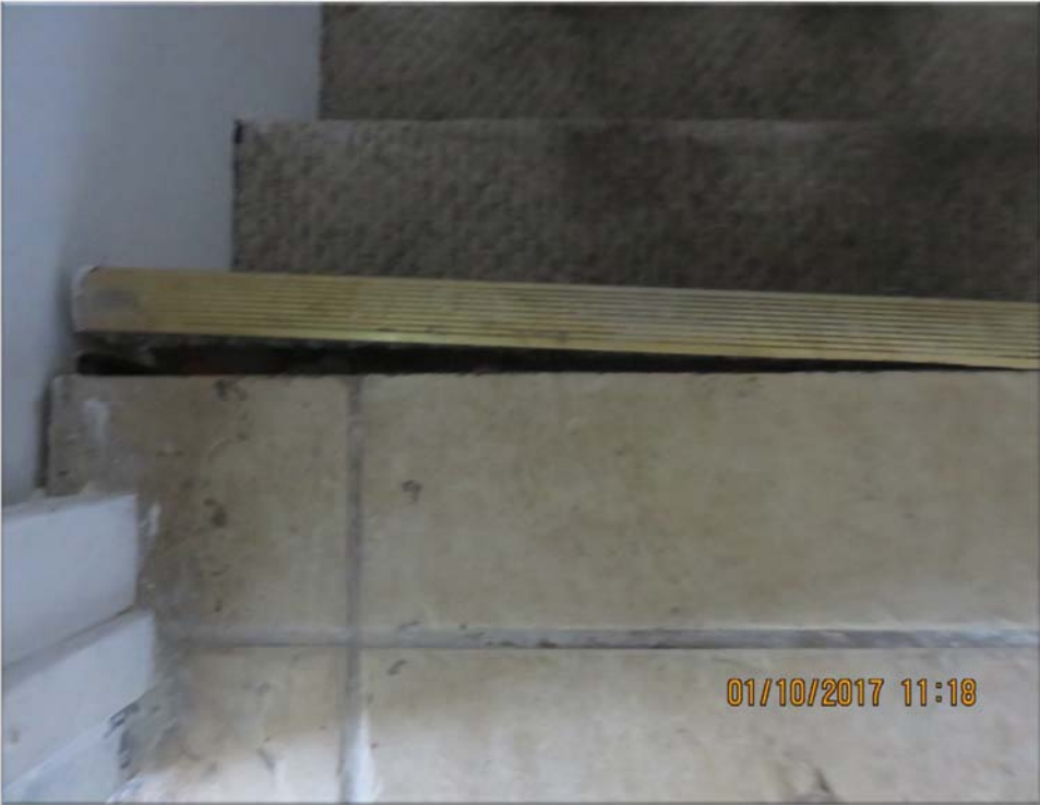
Property # OIG30: Broken threshold
