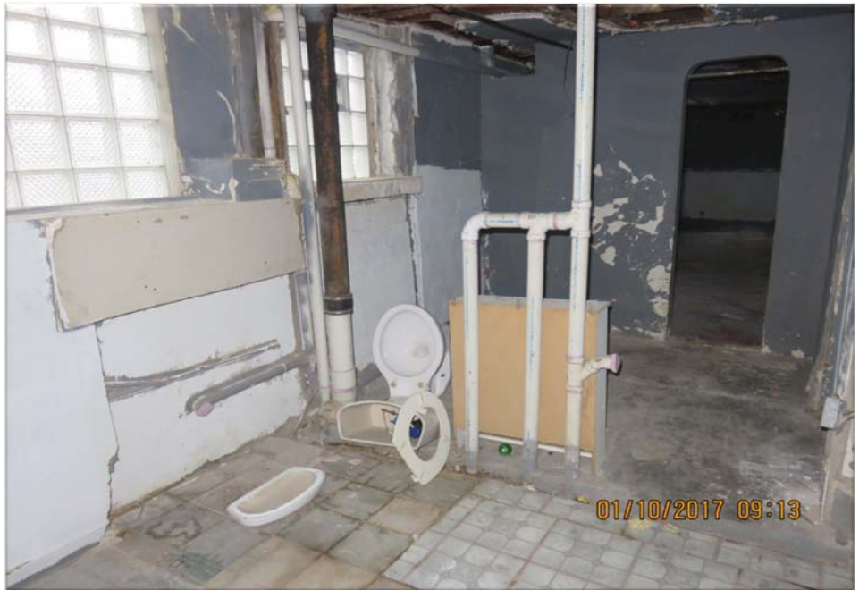
Property # OIG43: Debris in basement
