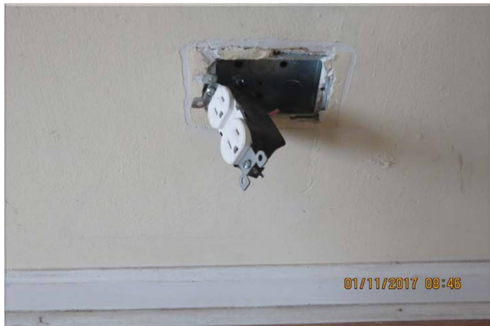
Property # OIG25: Broken outlet
