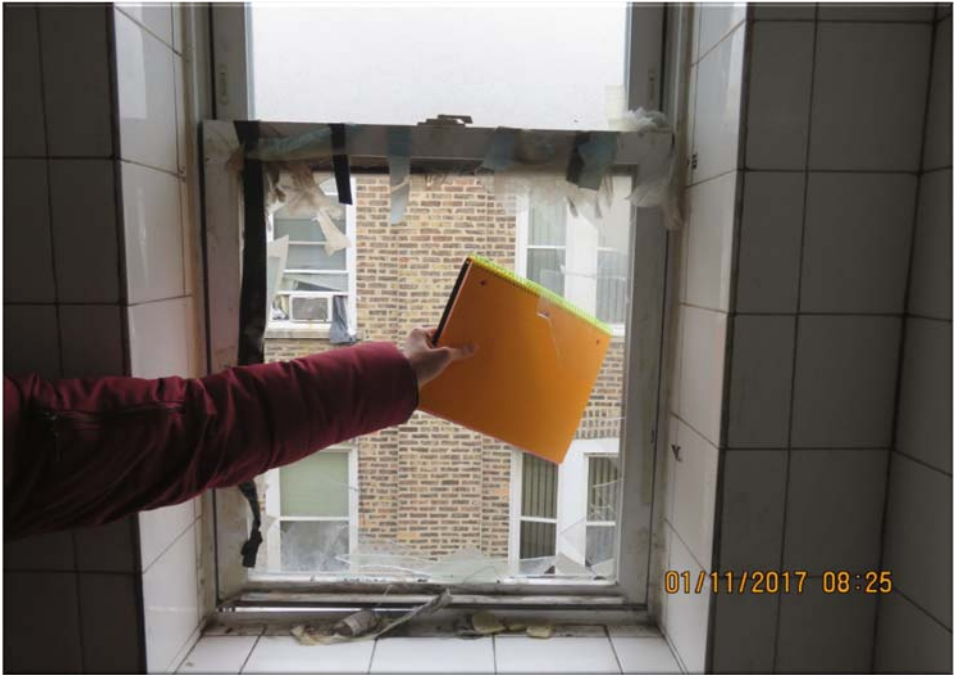
Property # OIG49: Broken window
