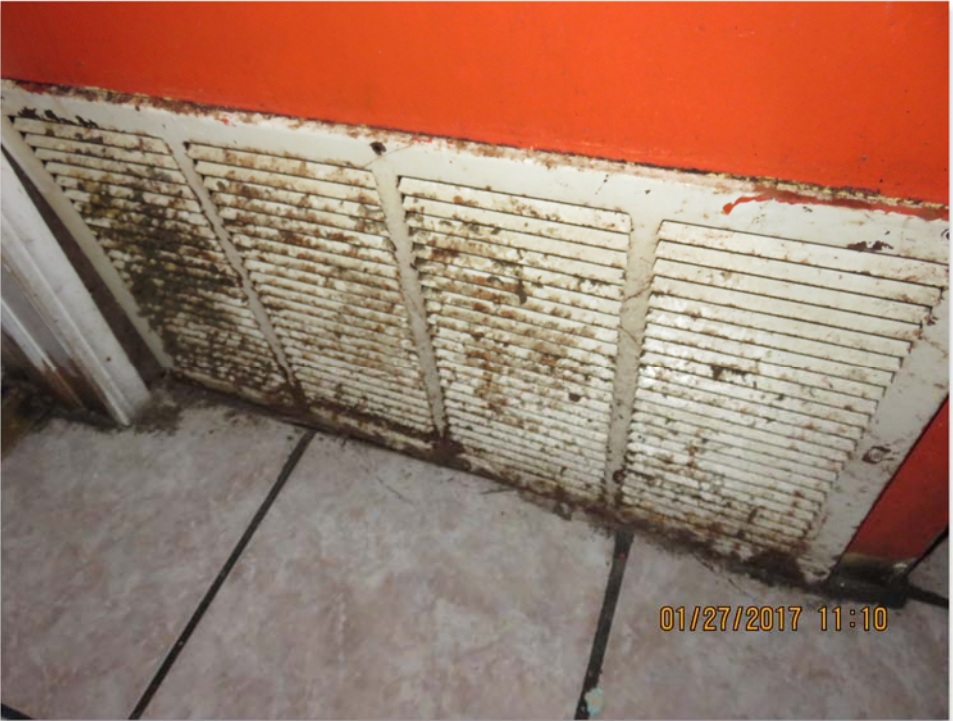
Property # OIG6: Dirty vent
