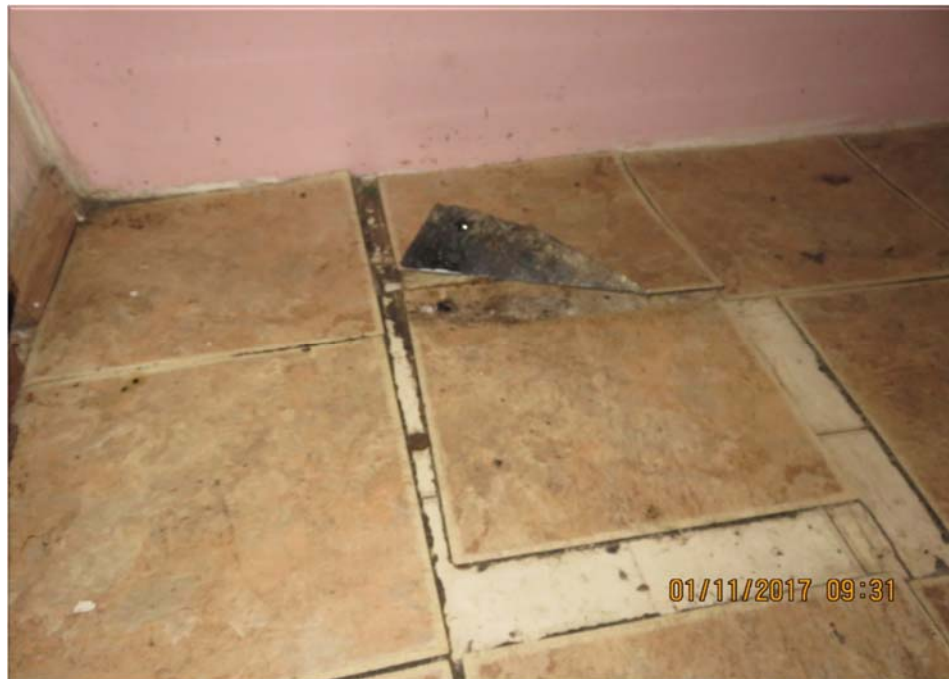
Property # OIG18: Tripping hazard
