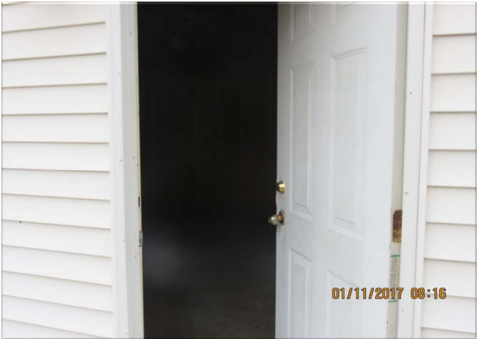
Property # OIG49: Unsecured garage door
