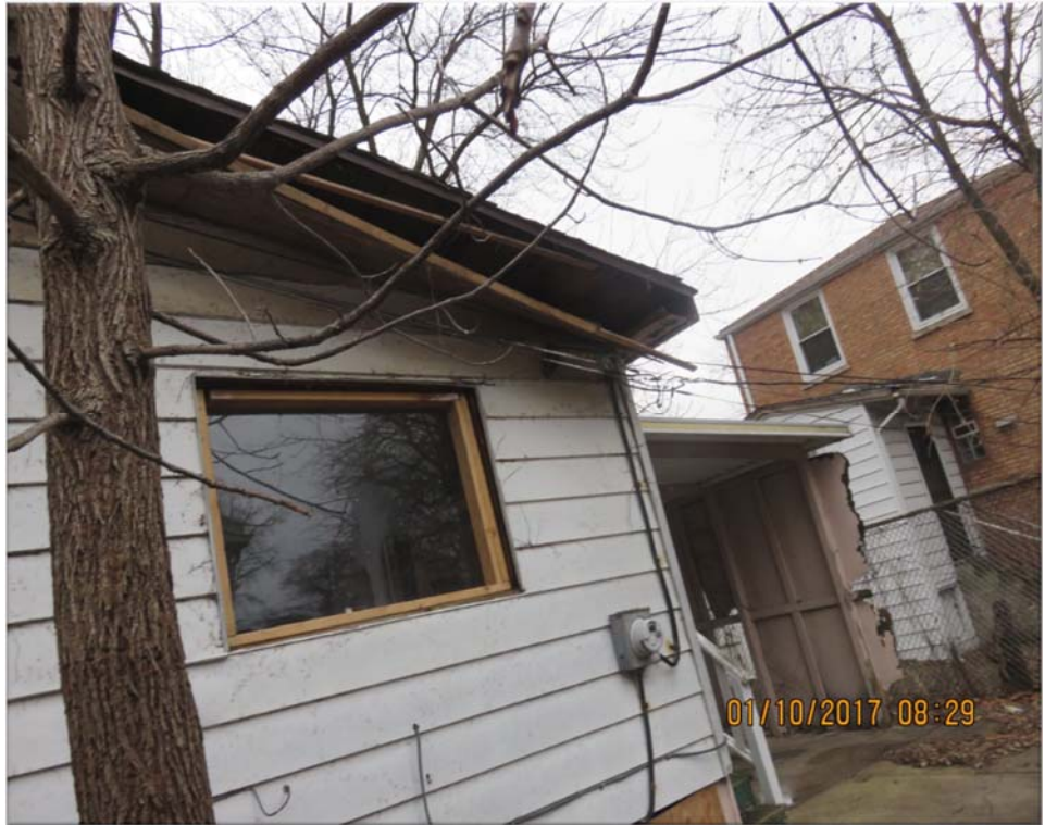
Property # OIG28: Unsecured roof board
