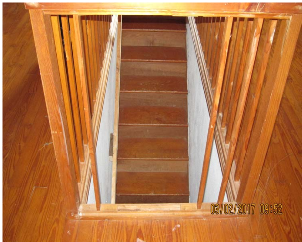
Property IS19: missing balusters in upstairs bedroom
