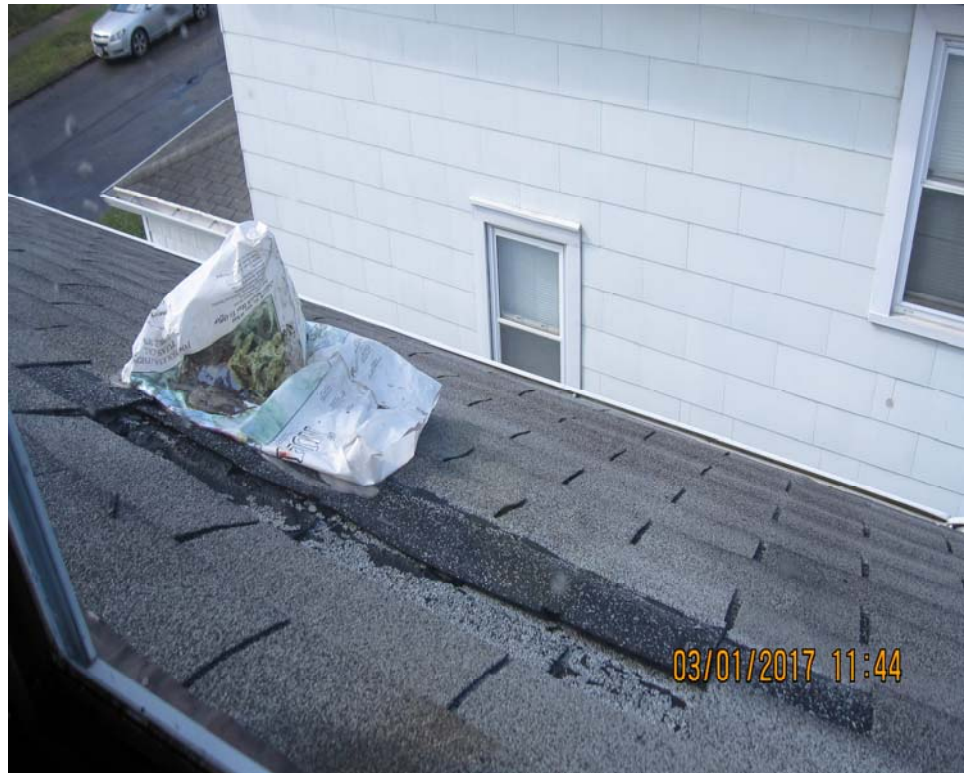
Property IS16: hole in roof covered by plastic bag – allowed water intrusion
