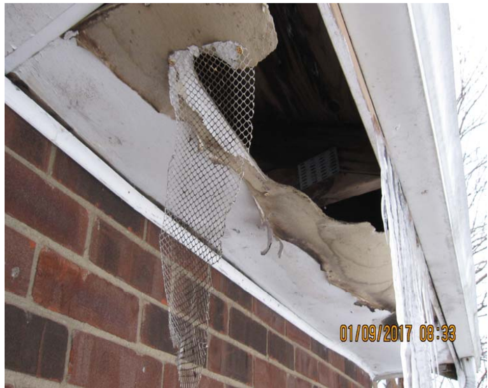
Property RI94: deteriorated rear soffit
