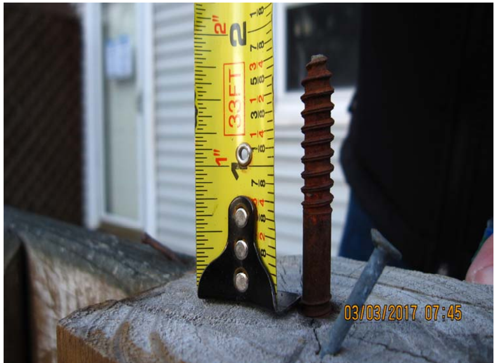
Property IS24: exposed screw and nail on rear deck
