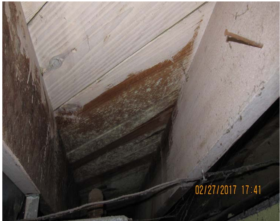
Property IS6: unmitigated mold in basement joists and subfloor
