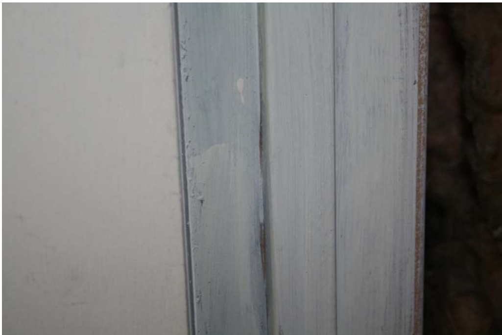
Smoke stains bleeding through paint - June 21, 2016
