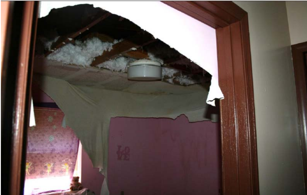
Ceiling collapse due to water damage - photographed on April 13, 2016
