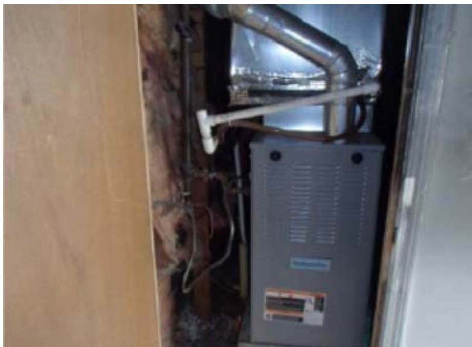
Insurance adjuster's photo showing smoke damaged insulation – July 10, 2013
