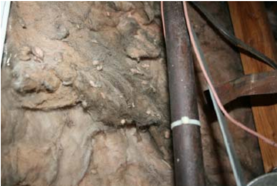
Smoke-damaged insulation not replaced after fire – photographed on June 21, 2016
