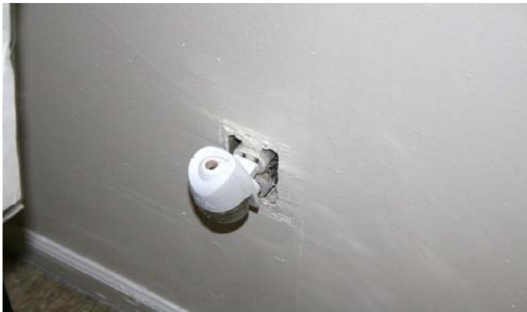
Poorly patched wall and receptacle cover not replaced after fire - photographed on June 21, 2016
