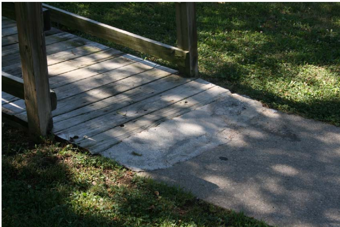
Concrete transition installed by maintenance - June 27, 2016
