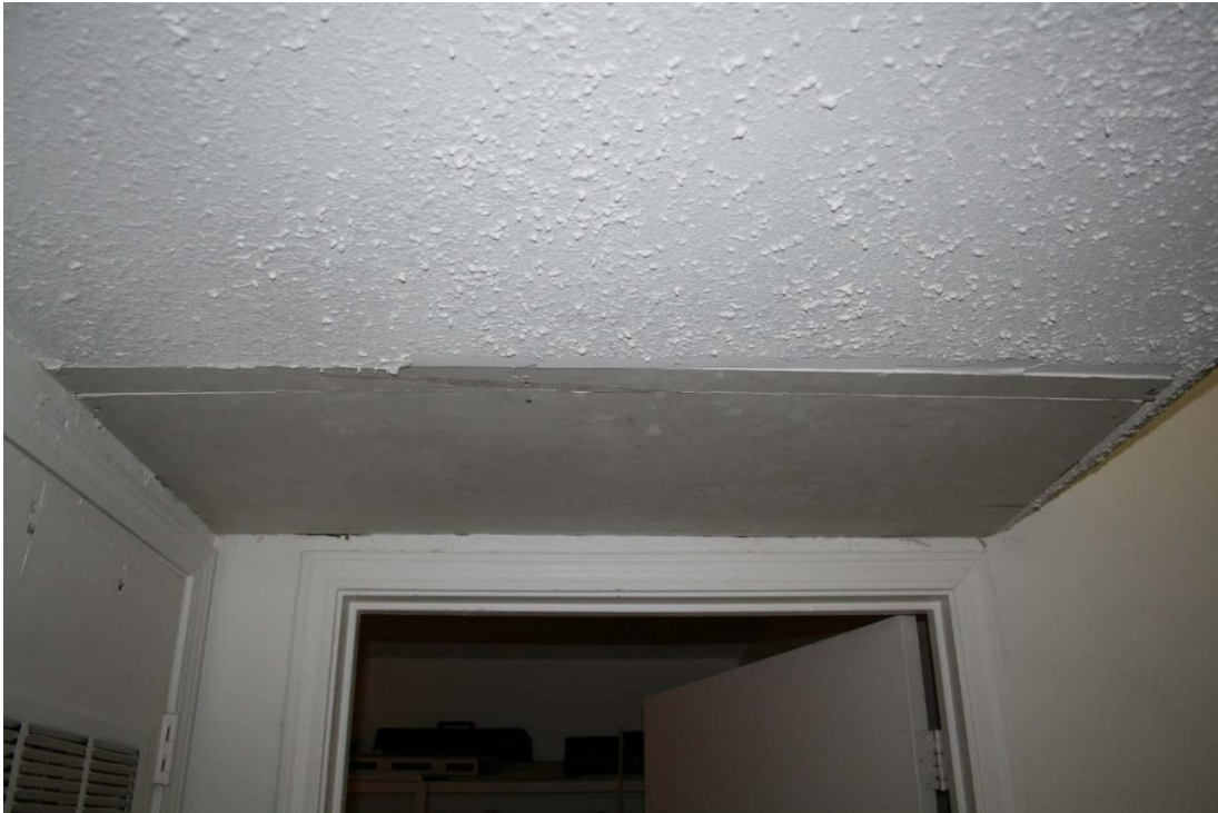
Poorly patched drywall - June 21, 2016
