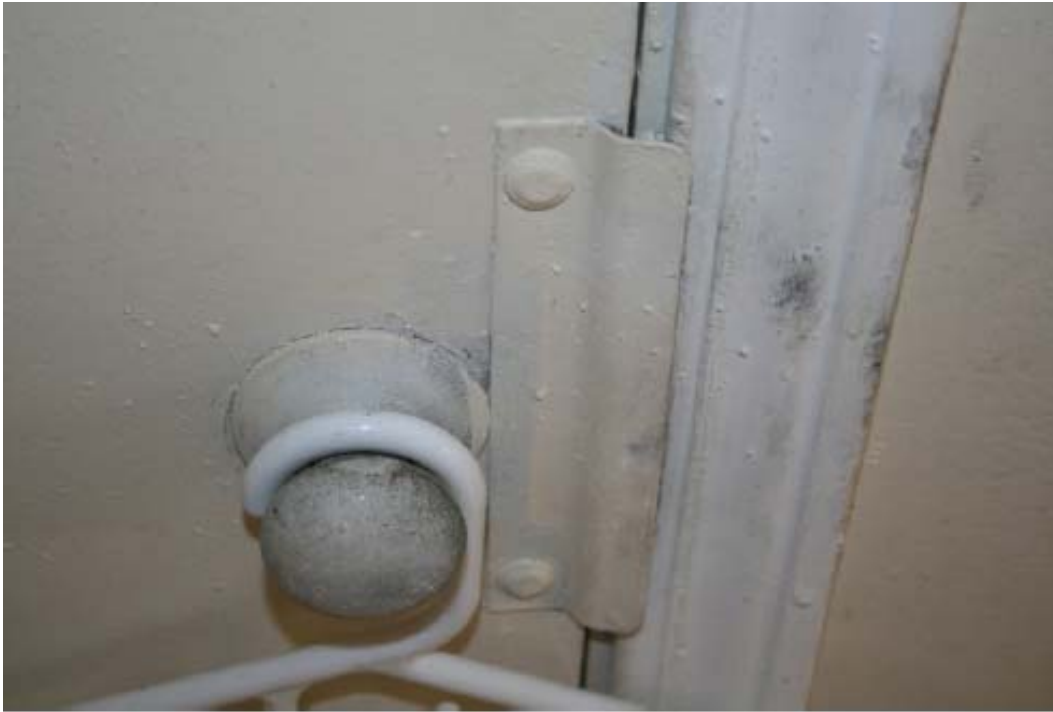
Soot from fire bleeding through paint - photographed on June 21, 2016
