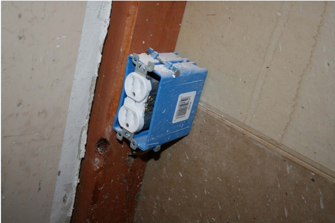
Outlet cover not installed - June 21, 2016
