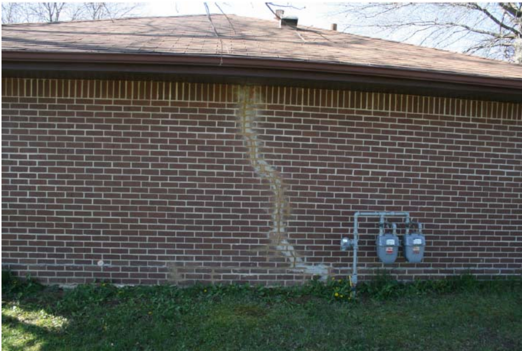
Poorly completed tuck-pointing - photographed on April 13, 2016
