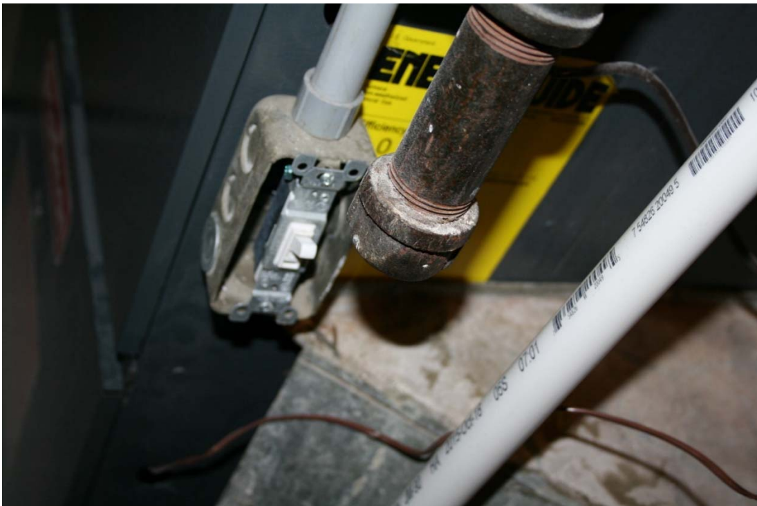
Switch cover not installed - June 21, 2016
