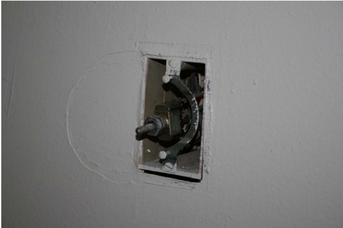
Switch cover not installed - June 21, 2016
