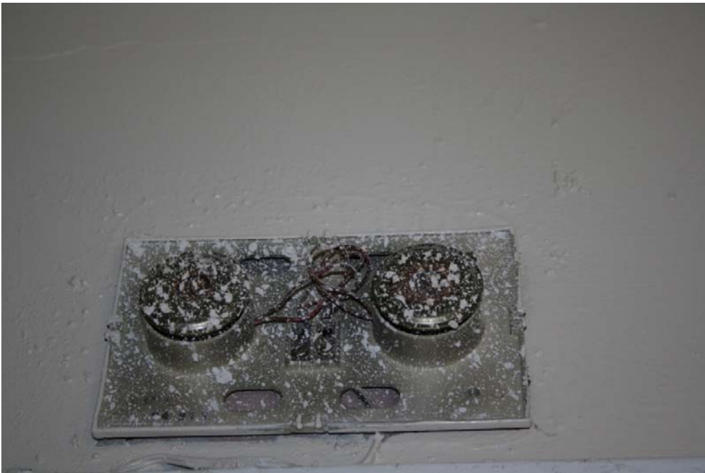
Fixture not removed prior to repainting - June 21, 2016
