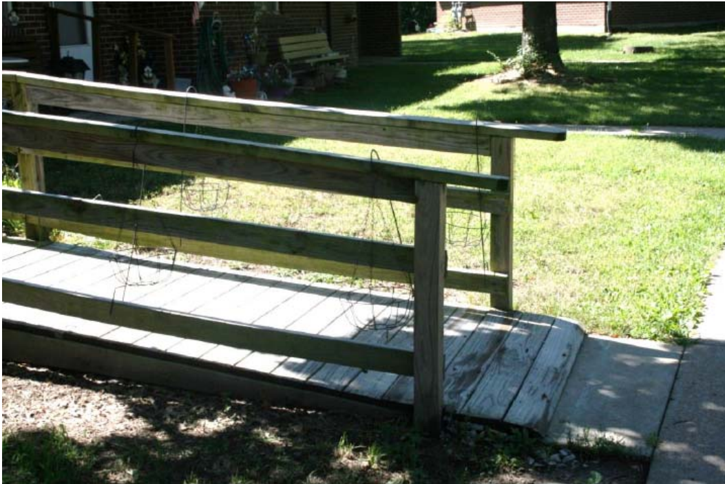
Concrete transitions to handicapped ramps not installed - photographed on June 27, 2016
