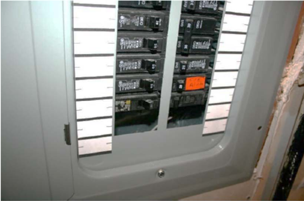
Missing breakers in breaker panel - photographed on June 21, 2016
