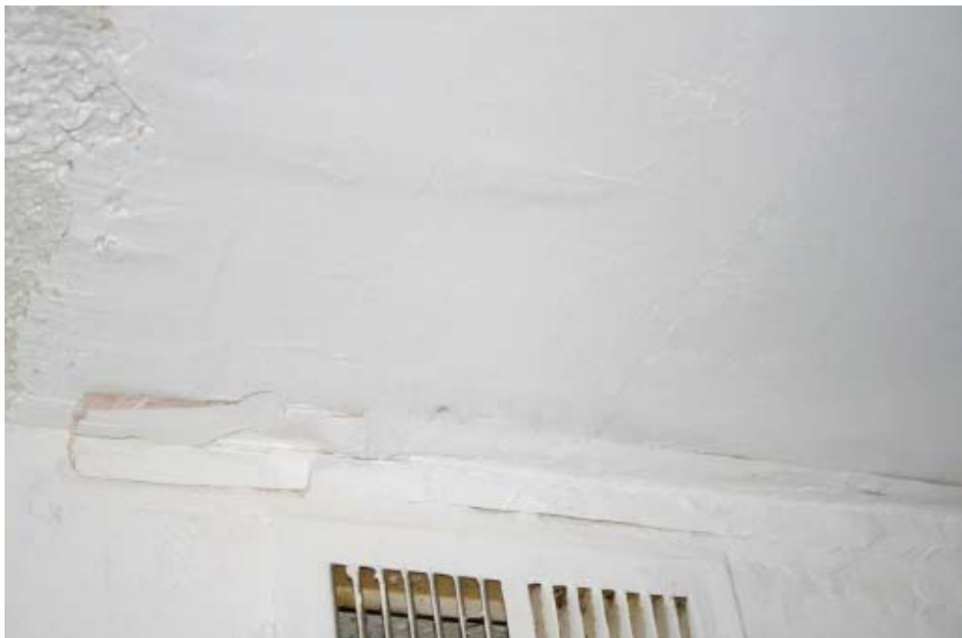
Sheetrock not properly finished - photographed on June 21, 2016
