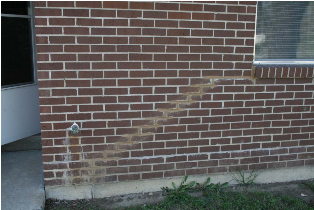
Poorly completed tuck-pointing - April 13, 2016
