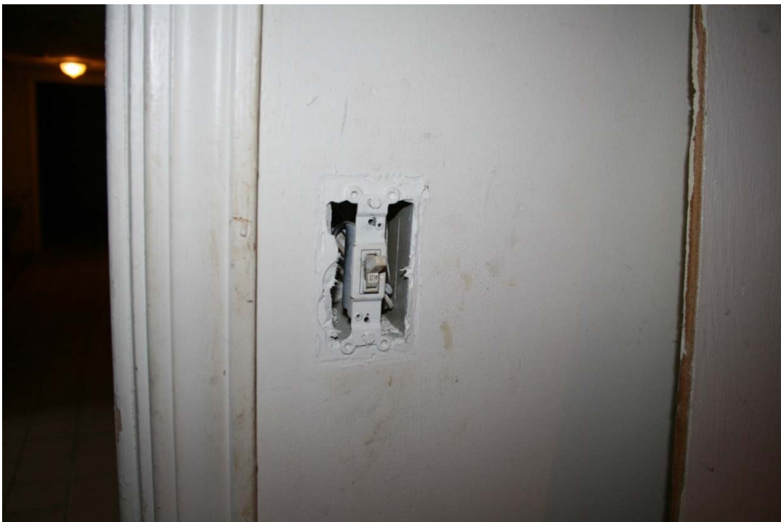
Switch cover not installed - June 21, 2016
