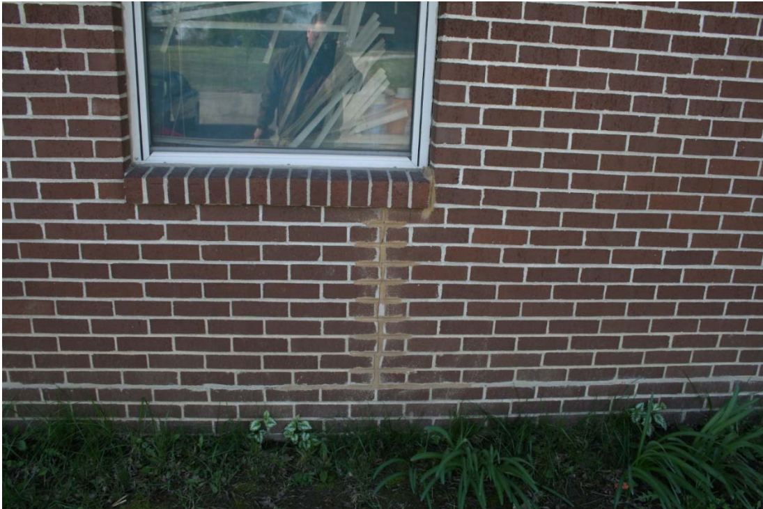
Poorly completed tuck-pointing - April 13, 2016
