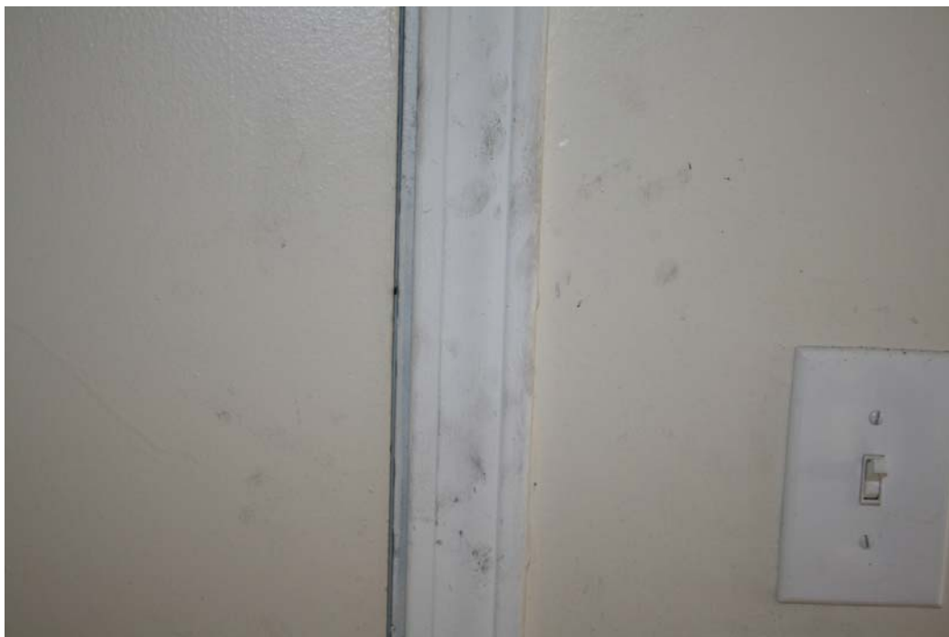
Smoke stains bleeding through paint - June 21, 2016
