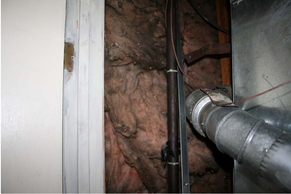
Smoke damaged insulation - June 21, 2016
