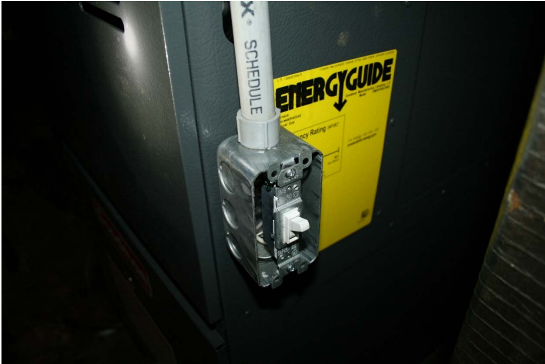
Switch cover not installed - June 21, 2016
