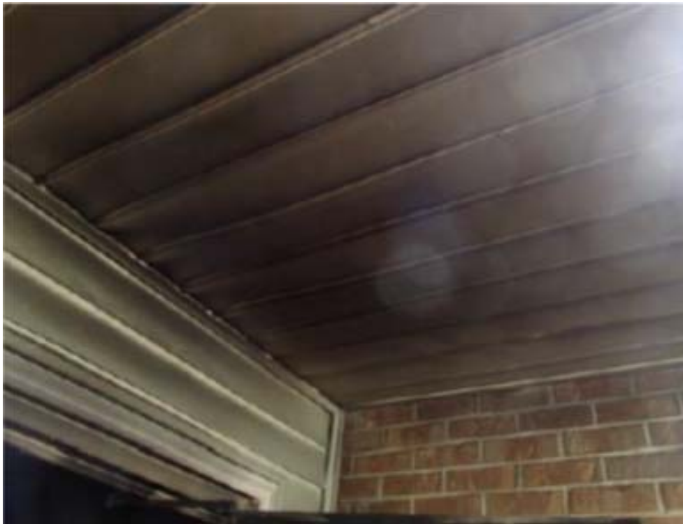
Insurance photo showing smoke damage to exterior vinyl – July 10, 2013
