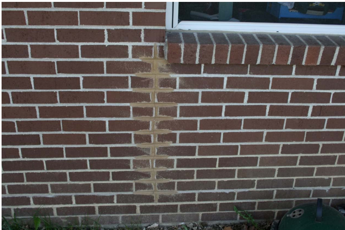
Poorly completed tuck-pointing - April 13, 2016
