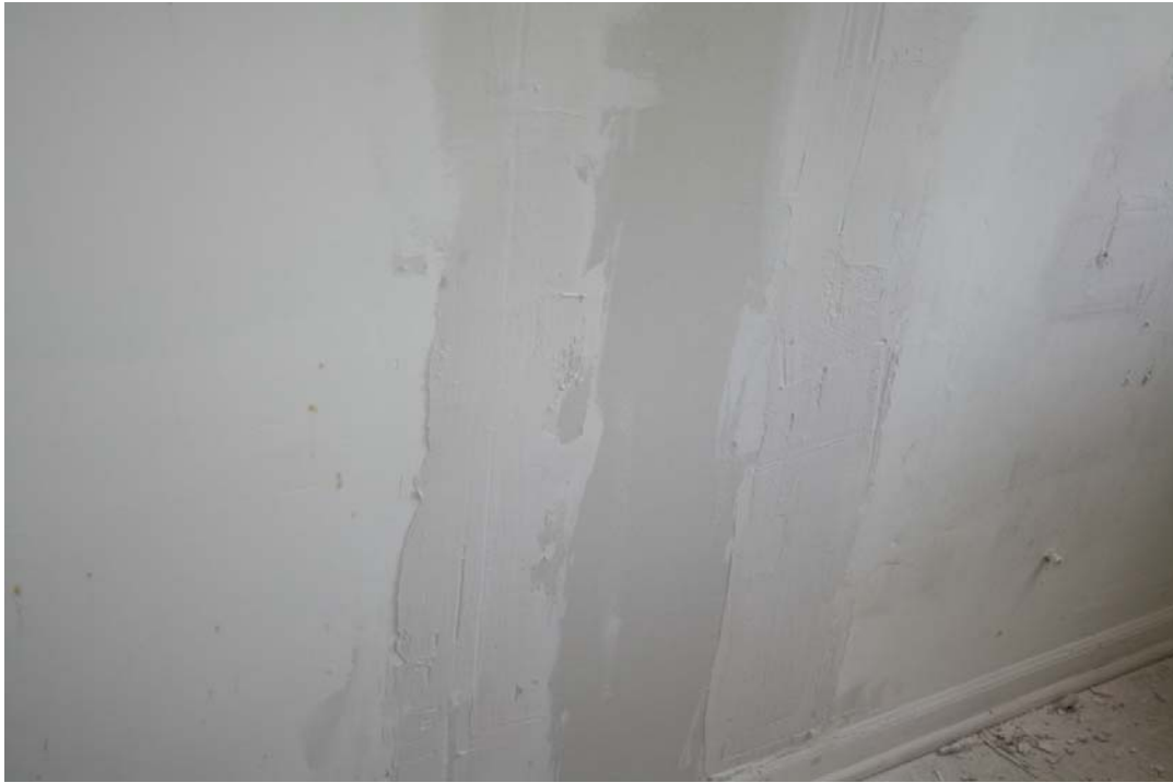
Poorly patched drywall - June 21, 2016
