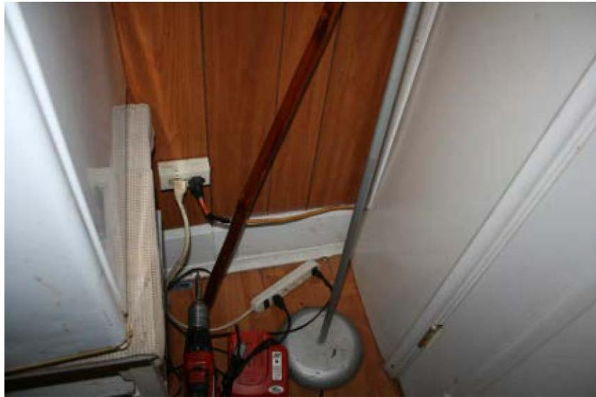
Inspection 64: There was an improper extension cord outlet connection. The extension cord ran through the wall of the closet to provide a receptacle. The Authority did not identify this violation during its June 13, 2017, inspection.
