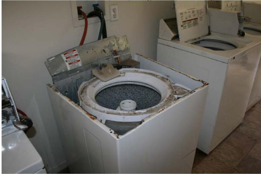
Inspection 34: There was a cutting hazard. The washing machine was missing its top, exposing sharp edges. The Authority did not identify this violation during its April 4, 2017, inspection.
