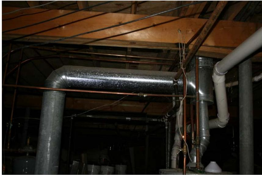
Inspection 39: An improperly sloped furnace pipe prohibited fumes from venting properly. The Authority did not identify this violation during its April 7, 2017, inspection.
