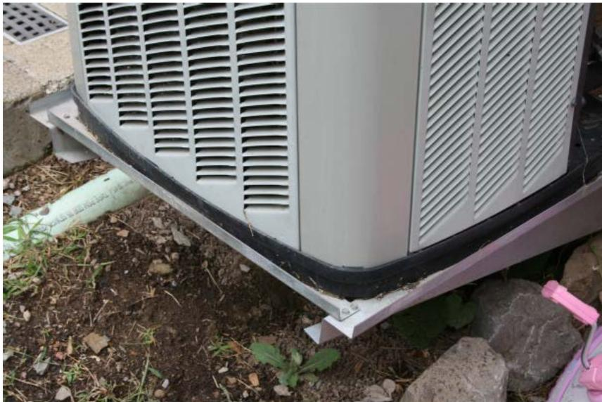
Inspection 54: The compressor unit was mounted on a metal support attached to the unit's exterior wall. The support had sharp edges and corners. The Authority did not identify this violation during its April 4, 2017, inspection.
