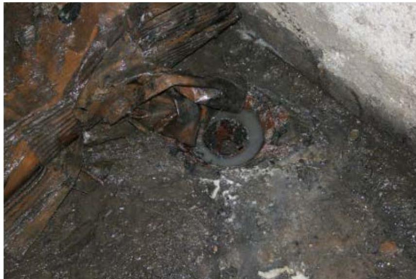
Inspection 25: The sewer cleanout in the basement was open and covered with pasteboard. Water and sewage were bubbling up. The Authority did not identify this violation during its May 17, 2017, inspection.
