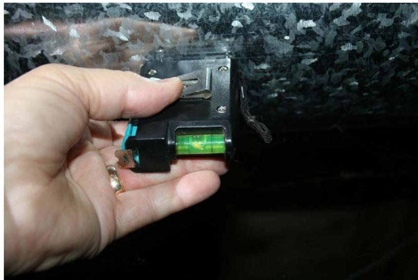
Inspection 39: This is an additional photo showing the improper slope of the furnace pipe. Because the pipe was not properly sloped, harmful fumes from the furnace could be prevented from exiting the building.
