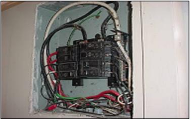
Breaker panel with no internal cover and with exposed electrical contacts, creating an electrical shock hazard. The deficiency was not reported by the authority during its February 26, 2007, inspection.
