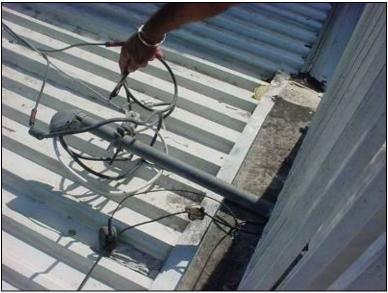
Main electrical connection resting above metal roof and within reach, creating an electrical shock hazard. The deficiency was not reported by the authority during its January 11, 2007, inspection.
