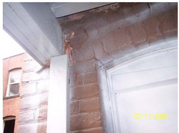
Exterior porch rotting and falling off support beam.
