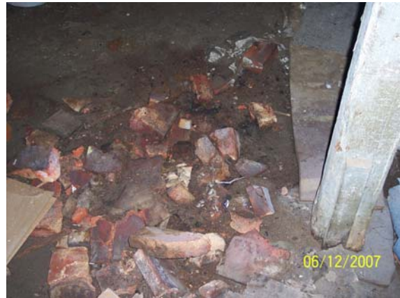
Basement floor torn up and debris on the floor causing a tripping hazard.
