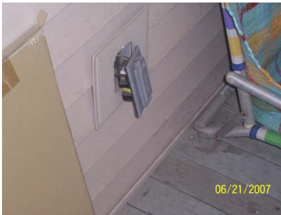
Outdoor electrical outlet that was not properly secured and exposed wires.
