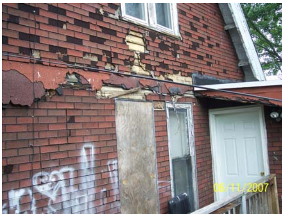
Exterior siding falling off the building.
