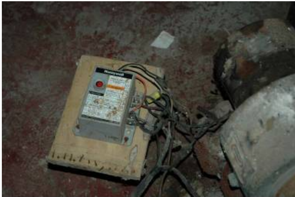
Inspection #29: There are exposed contacts on a furnace controller near the basement floor. This violation was not identified during the Authority's April 26, 2007, inspection.
