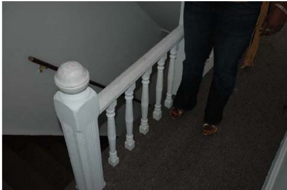
Inspection #47: The banister protecting the stairway opening on the third floor is only 23 inches from the floor and insufficiently high for protection. Also, the handrail on the stairway to the third floor stops three steps short of the top. Neither of these violations was identified during the Authority's July 25, 2007, inspection.
