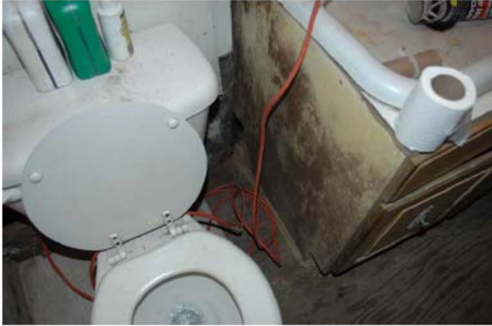
Inspection #23: Mold is present in the basement bathroom on the vanity and wall. This violation was not identified during the Authority's June 29, 2007, inspection.
