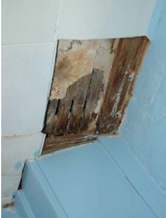
Inspection #23: Damage to plaster and missing ceiling tiles in the back bedroom on the second floor were caused by a leak in the roof of the adjacent abandoned unit. The violation was not identified during the Authority's June 29, 2007, inspection.
