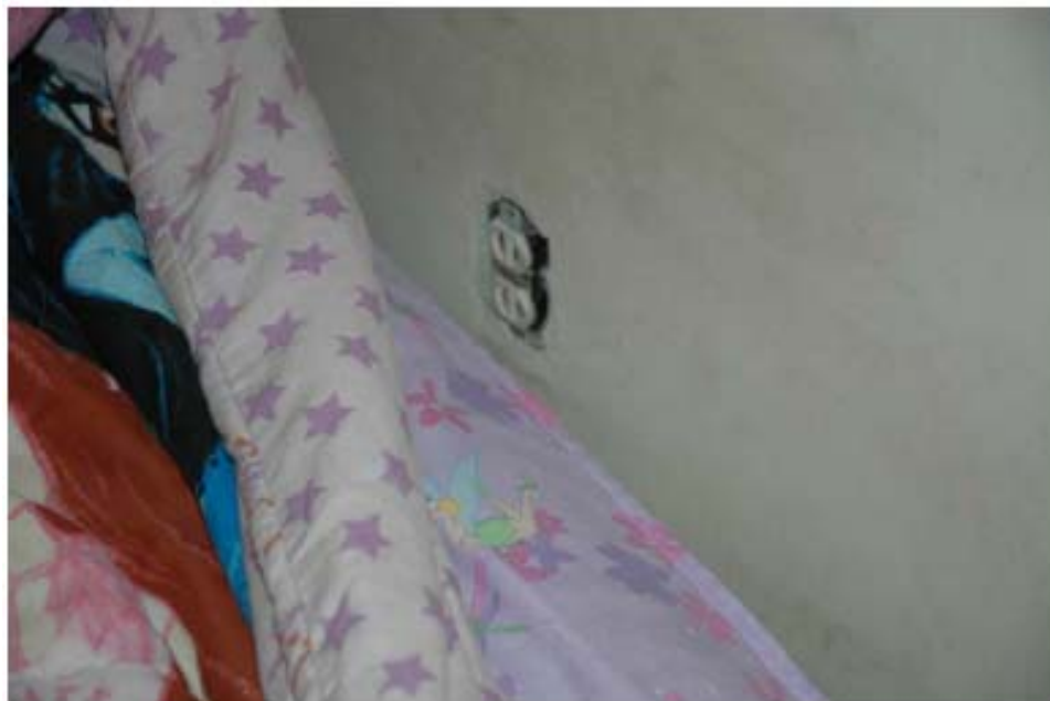
Inspection #38: The cover plate is missing from the left/rear bedroom wall outlet. This violation was not identified during the Authority's April 26, 2007, inspection.
