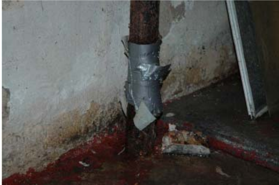
Inspection #29: A leaking drain pipe from the kitchen is wrapped with duct tape in failed attempts to stop the leak. This violation was not identified during the Authority's April 26, 2007, inspection.
