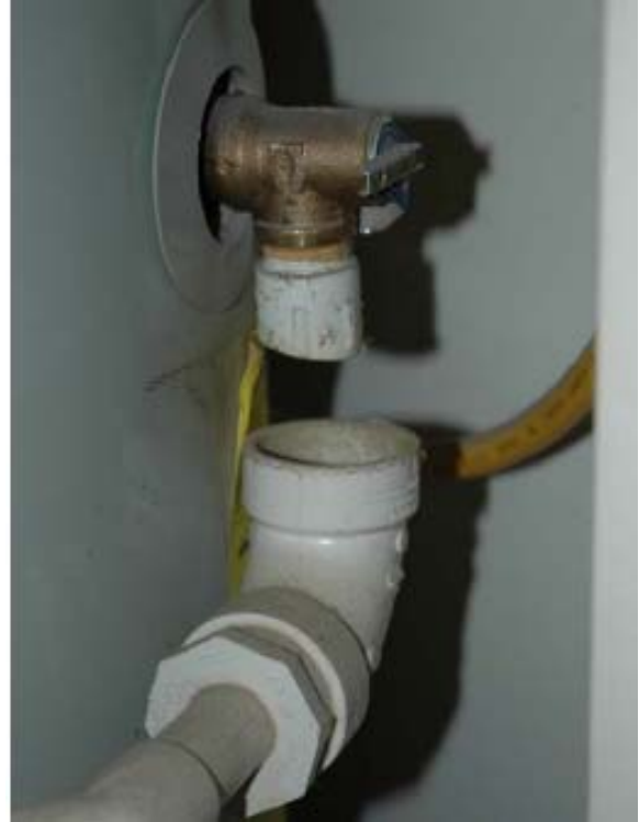
Inspection #52: There is an unacceptable discharge pipe on the water heater's pressure relief valve that leaves a gap through which escaping steam can scald a tenant. The pipe needs to be continuous to within a minimum of six inches off the floor. This violation was not identified during the Authority's July 5, 2007, inspection.
