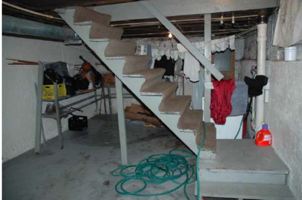
Inspection #35: There is a loose carpet on the basement stairs, and a guardrail is needed on the open side of the staircase. This violation was not identified during the Authority's April 26, 2007, inspection.
