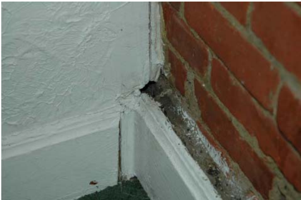
Inspection #47: A mouse hole and droppings are above the baseboard in the dining room. This violation was not identified during the Authority's July 25, 2007, inspection.
