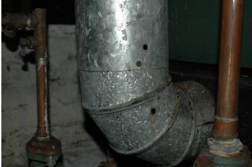
Inspection #16: Holes in the boiler's flue allow carbon monoxide to enter the basement. This violation was not identified during the Authority's October 25, 2007, inspection.
