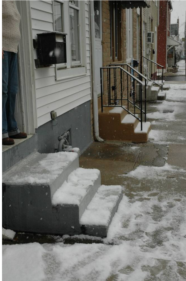
Inspection #8: The front stoop has no handrail. (Note adjacent stoops have handrails.) This violation was not identified during the Authority's August 17, 2007, inspection.
