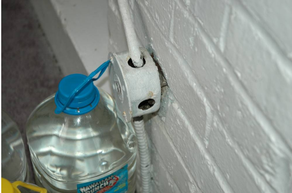
Inspection #14: A junction box in the rear porch has a hole and a wire that is not secured with a wire connector. This violation was not identified during the Authority's August 14, 2007, inspection.
