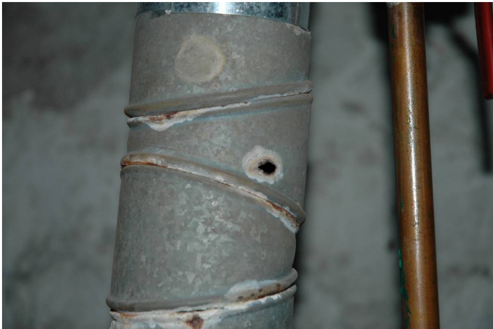
Inspection #53: A hole in the water heater's flue allows carbon monoxide to enter the basement. This violation was not identified during the Authority's October 29, 2007, inspection.
