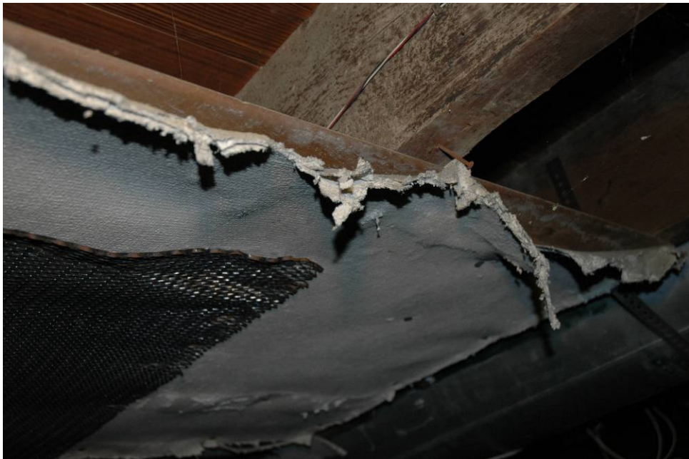
Inspection #30: An asbestos sheet on the basement ceiling has a frayed edge. This violation was not identified during the Authority's September 13, 2007, inspection.
