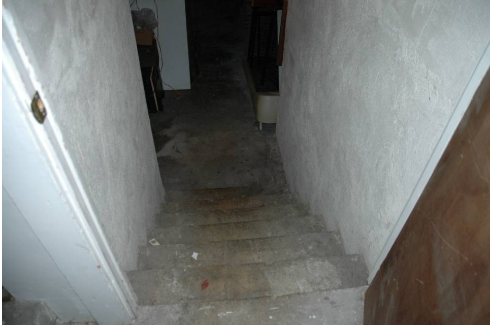
Inspection #25: The stairway to the basement does not have a handrail. This violation was not identified during the Authority's September 11, 2007, inspection.
