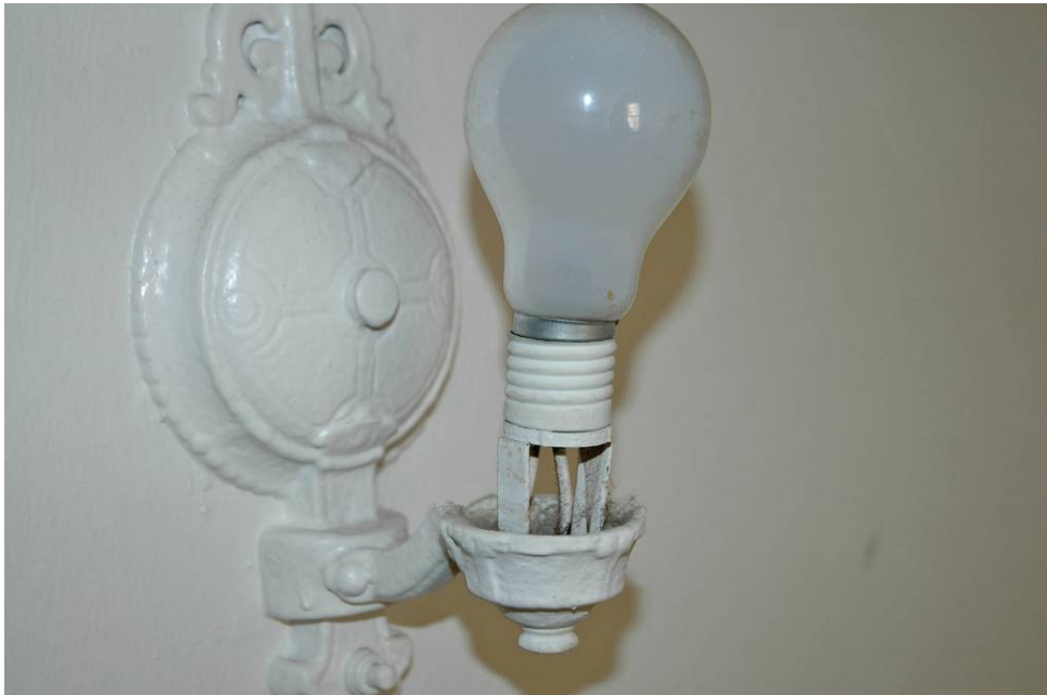
Inspection #38: A wall lamp on a third floor stairway wall is missing the insulator over the socket, exposing electrical contacts. This violation was not identified during the Authority's August 27, 2007, inspection.
