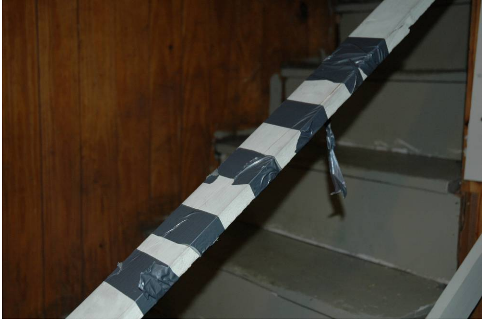
Inspection #16: Broken 2x4 makeshift handrail needs to be replaced and be constructed with an intermediate support. This violation was not identified during the Authority's October 25, 2007, inspection.
