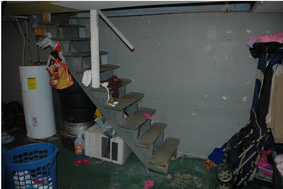
Inspection #32: The handrail at the basement stairway stops too short from the bottom of the stairs. This violation was not identified during the Authority's August 14, 2007, inspection.
