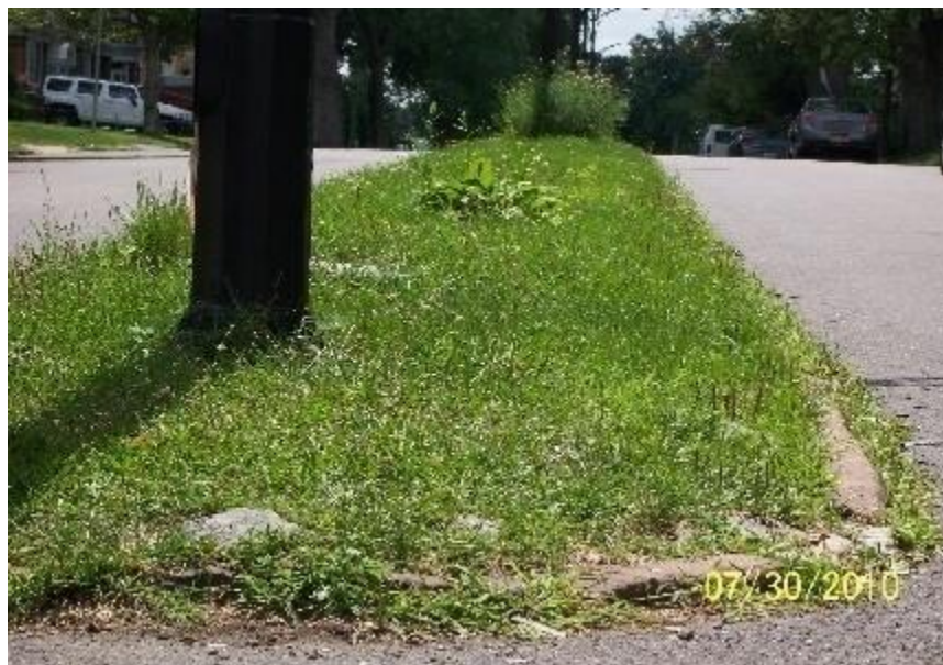
The Agency reimbursed the City using CDBG funds for a median curb replacement project on Academy Road that was not done. The picture above illustrates that the median curb was not replaced.
