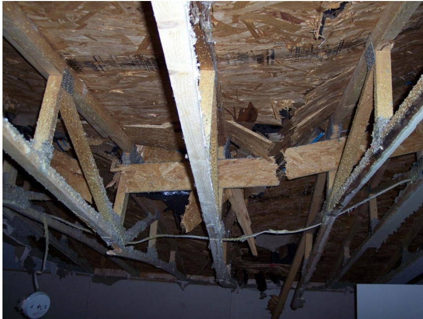
Figure 11: Interior view of the damaged manufactured home showing the shattered roof, joists, and rafters
