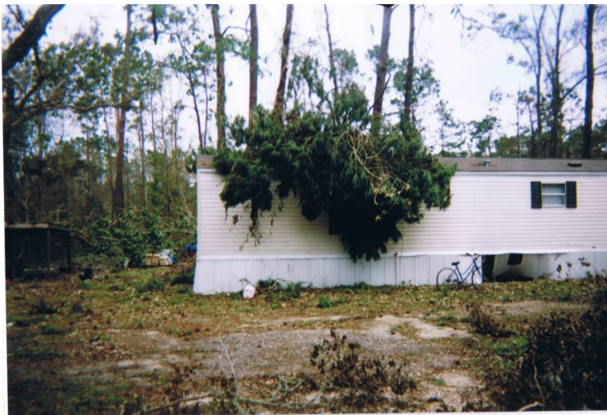
Figure 10: Uninsured manufactured home damaged by Hurricane Ike
