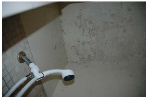
The ceiling above the shower stall in the second bathroom has mold and peeling paint.
