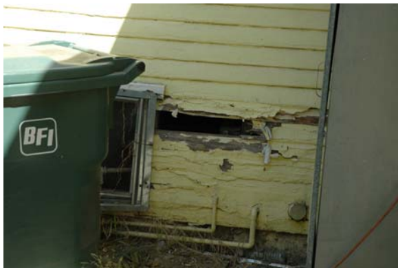
There is rotting siding and a hole in the back wall of the house.
