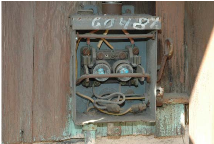
An electric panel had no cover, leaving electrical contacts exposed.
