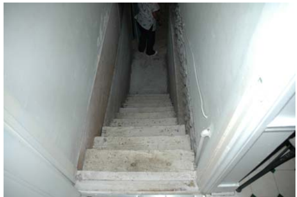
The stairway to the basement has no handrail.
