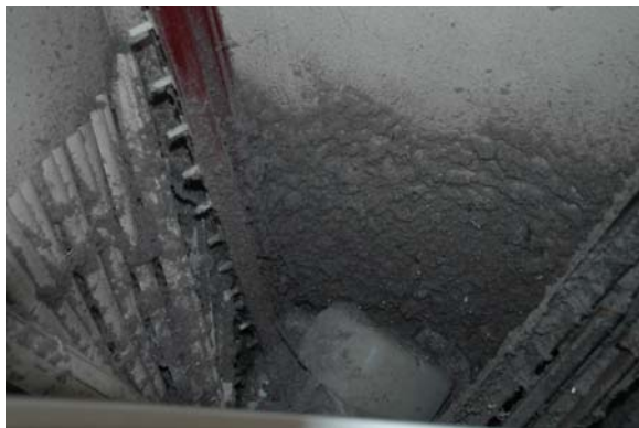
Lint collected behind the dryer, which is not connected to a vent, creating a fire hazard.
