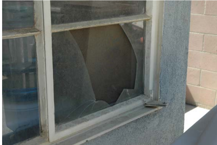
A broken glass pane on a kitchen window poses a cutting hazard.
