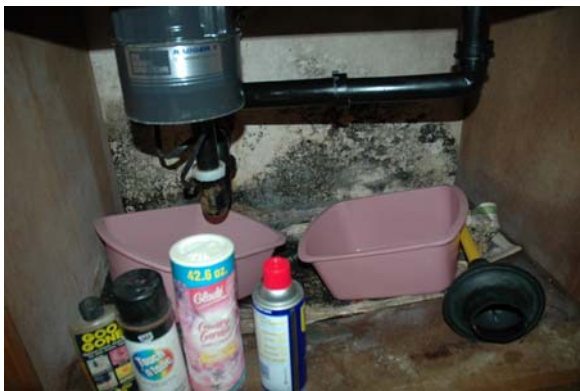
The leaking sink drain pipe has caused damage and mold on the wall and cabinet bottom panel.
