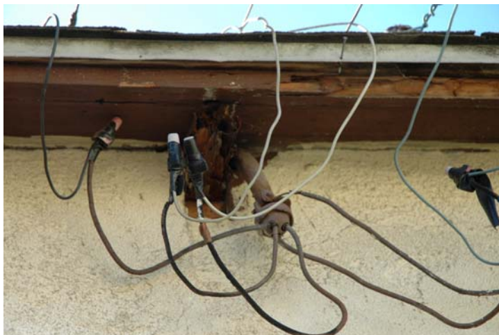
Improper wires were used to replace old wiring to bring power from the house to the garage. These wires need to be inside a conduit or other type of shielding and should not be exposed.
