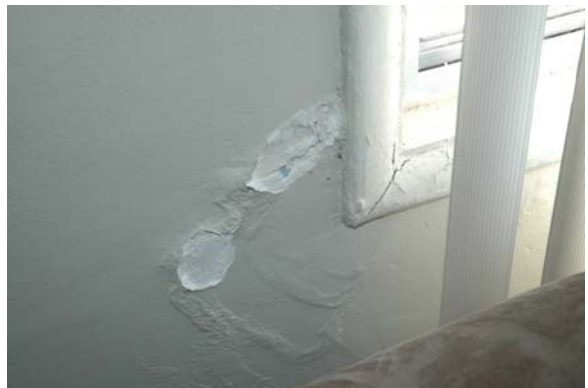
There is peeling paint on the living room wall.
