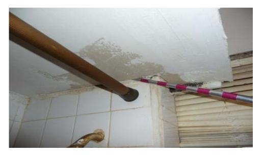
During an inspection of sample unit # 29 conducted on February 4, 2008, this unit's bathroom had what appears to be faulty ceiling repair work in
