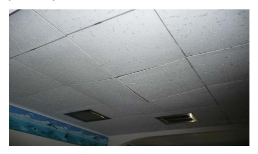
During an inspection of sample unit #8 conducted on January 30, 2008, this unit's bathroom had a buckling and bulging ceiling.
