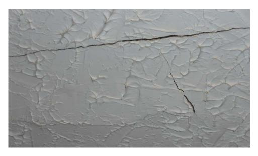
During an inspection of sample unit #51 conducted on February 12, 2008, the rear center bedroom of this unit had several cracks in the ceiling.
