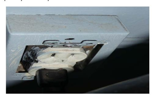
During an inspection of sample unit #29 conducted on February 4, 2008, this unit's bedroom had an electrical outlet with a missing face plate, which can be hazardous.
