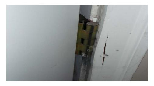
During an inspection of sample unit #34 conducted on February 5, 2008, this unit's main entry door had the hinges and hinge pins on the exterior of the door, and a split frame, all of which compromised the security of the unit.
