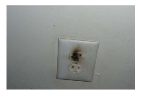
During an inspection of sample unit # 26 conducted on February 04, 2008, this unit's living room contain a socket with faulty electrical problems for which the tenant states caused sparks when an item is plugged into it.
