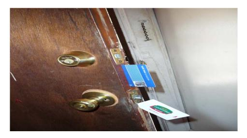
During an inspection of sample unit #11 conducted on January 30, 2008, this unit's main entry door was split, and it had a double key lock, which could become a safety issue during a fire.
