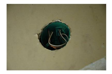
Project #3836: The 2<sup>nd</sup> floor left/rear bedroom ceiling fan was improperly connected and has a short in it.
