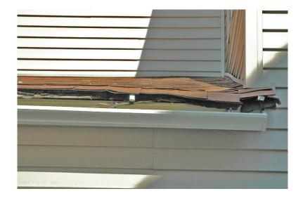
Project #3874: The edge of the roof on the left side of the house shows wood deterioration.
