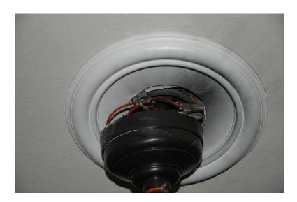
Project #3869: The junction box on the basement ceiling is open and has exposed wires and connections.
