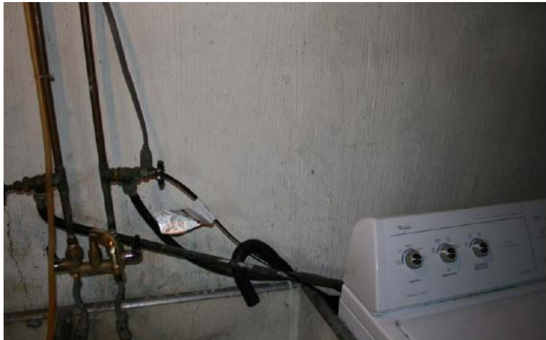
Inspection #8: Washer outlet needs grounded outlet away from faucet. This violation was not identified during the Authority's December 24, 2007, inspection.
