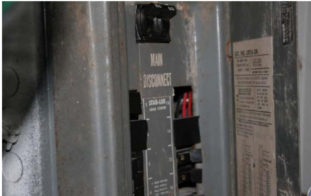
Inspection #2: Plugs were missing on breaker box. This violation was not identified during the Authority's December 5, 2007, inspection.
