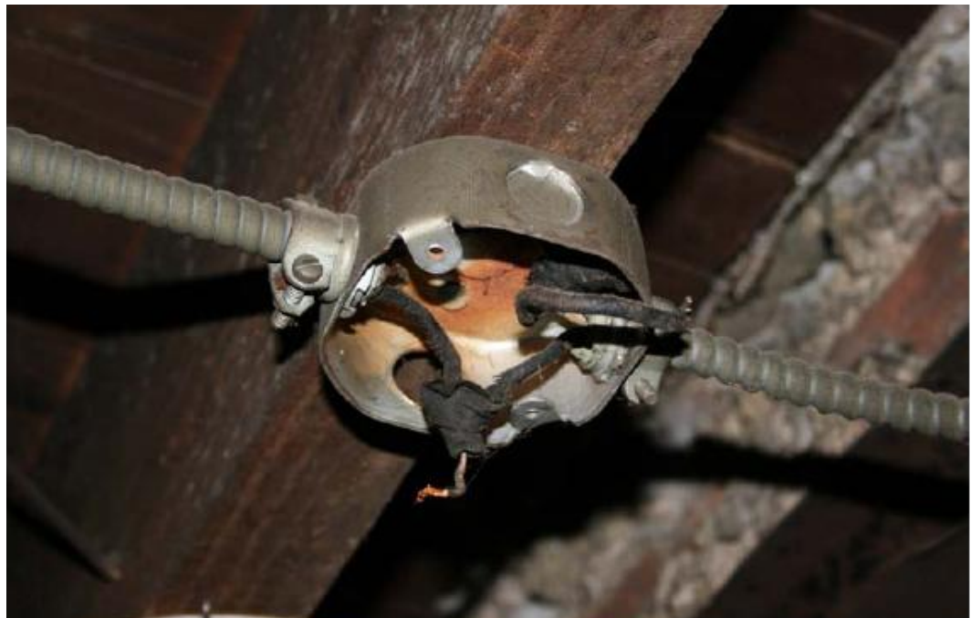
Inspection #31: Junction did not have wire nut and a cover to protect from injury. This violation was not identified during the Authority's October 16, 2007, inspection.
