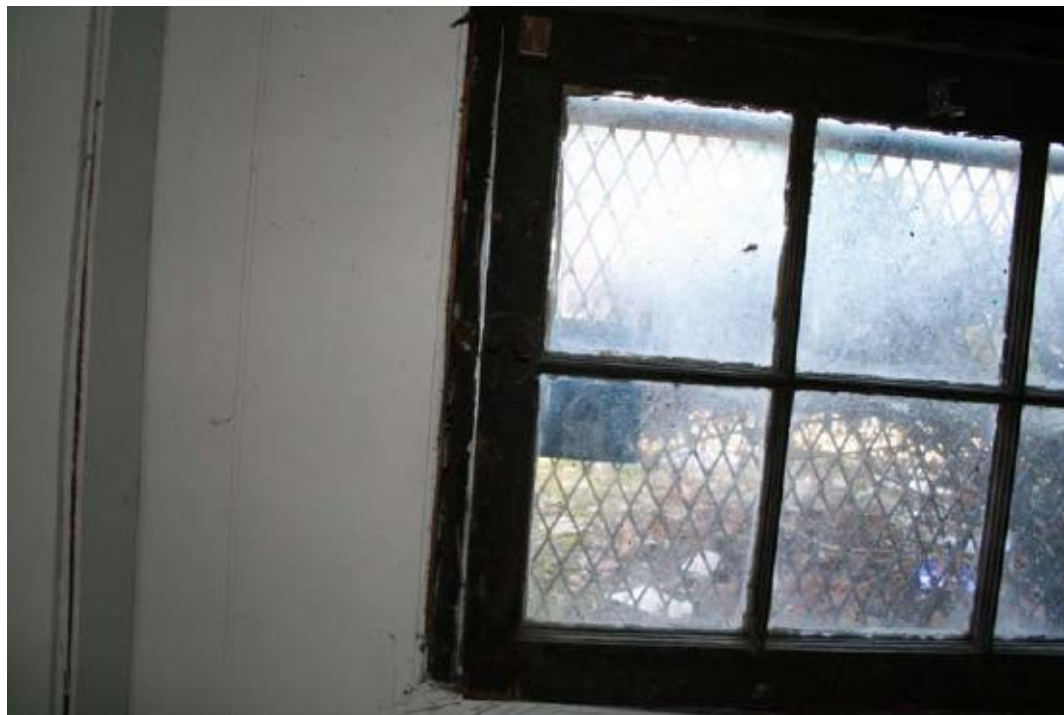
Inspection #21: The basement window will not close. This violation was not identified during the Authority's December 5, 2007, inspection.
