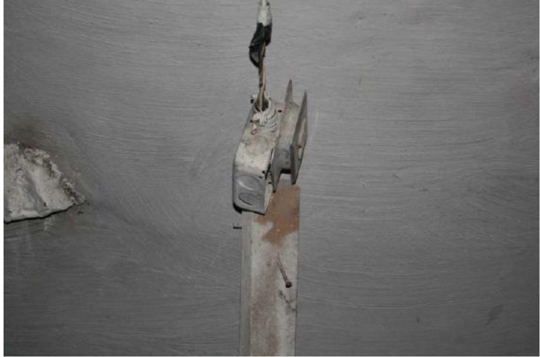
Inspection #19: Outlet was loose from ceiling with open ground. This violation was not identified during the Authority's November 30, 2007, inspection.
