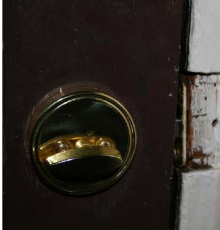
Inspection # 7: The striker plate on the rear basement door was loose and broken out. This violation was not identified during the Authority's November 15, 2007, inspection.
