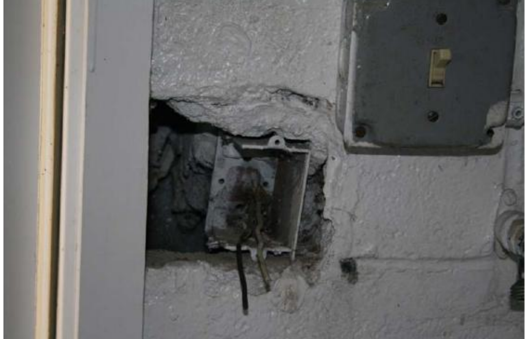
Inspection #57: Exposed wiring was found in community area of unit. This violation was not identified during the Authority's October 16, 2007, inspection.
