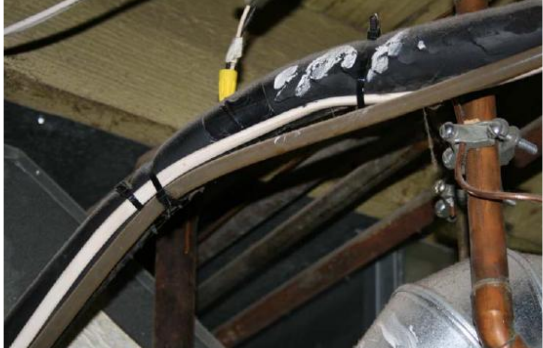
Inspection #40: Hot wire needs to be terminated in junction box and removed from conduit. This violation was not identified during the Authority's October 30, 2007, inspection.
