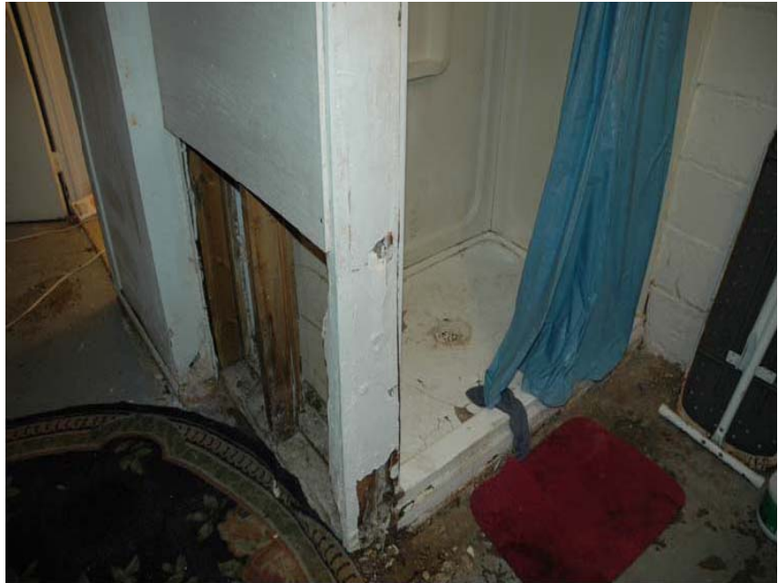
Unit #12141: Damaged and missing wall sections caused by plumbing leaks.
