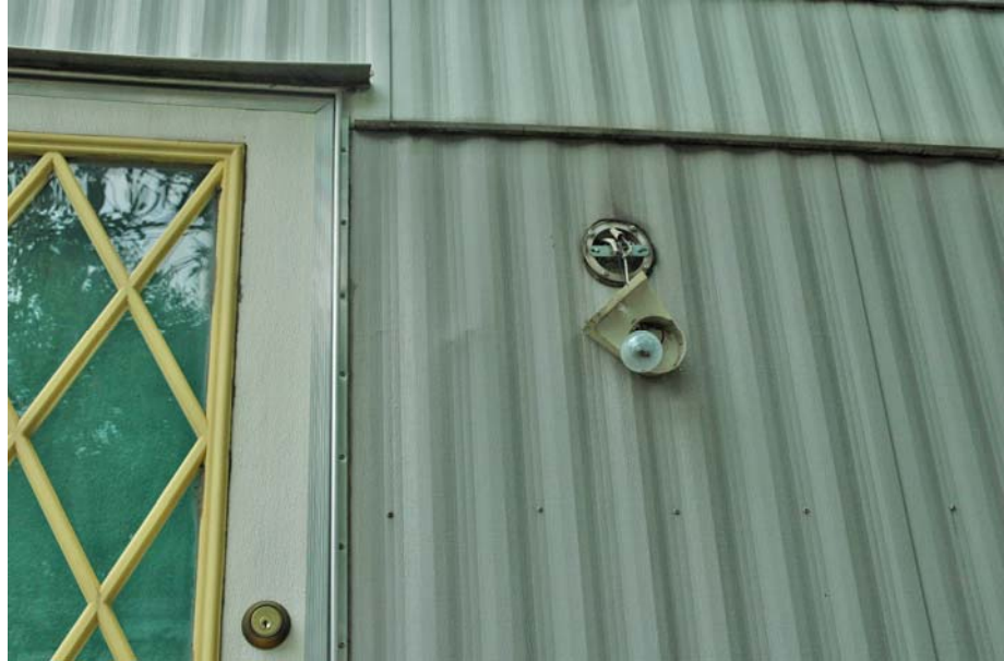
Unit #1: Exterior wall lamp next to the laundry room door hanging from its wires.
