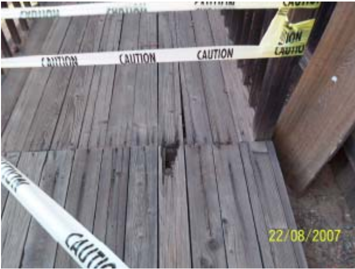
Back yard deck (rotten and cordoned off)
