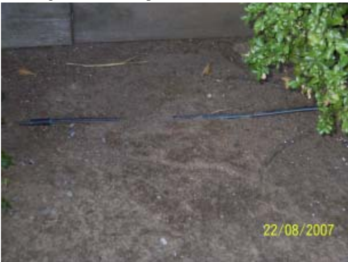
Irrigation hoses exposed from erosion
