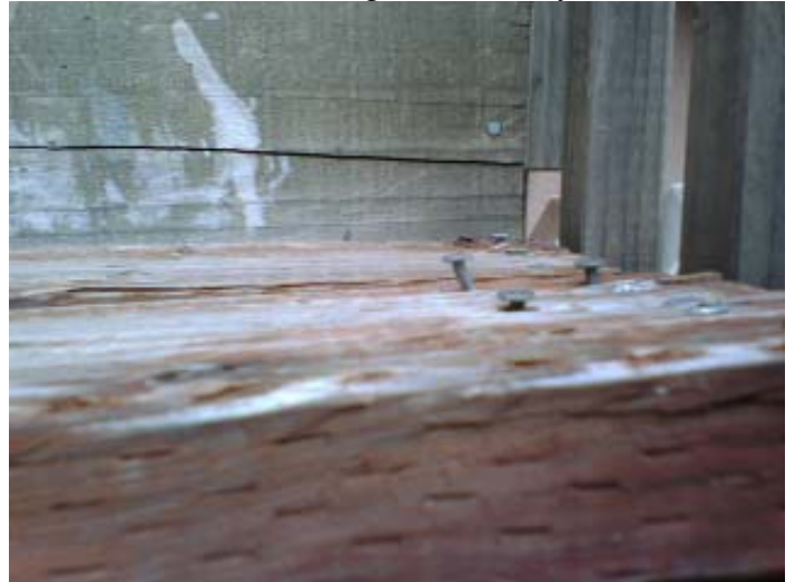
Cracked stairs leading to the back yard
