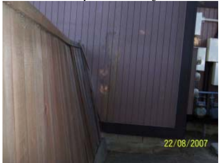
Back yard fence leaning
