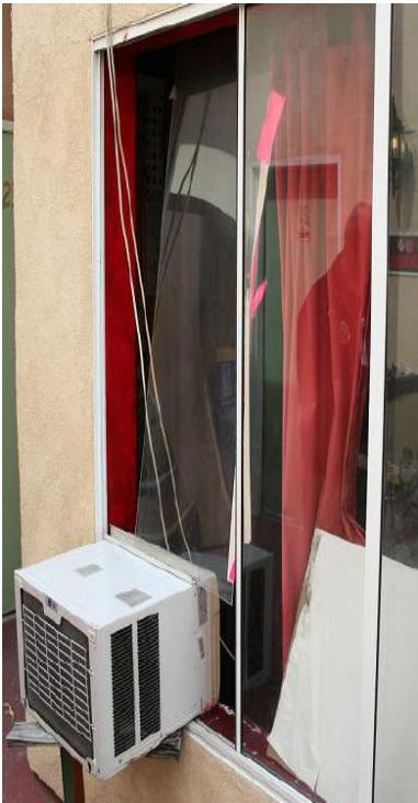
Assessor parcel numbers 5028001028 and 5163013009: Broken glass raises concerns for safety of tenants and poses a cutting hazard.
