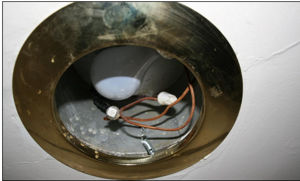
Inspection V54274: There are exposed wires in the recessed light fixture. This violation was not identified during the Authority's December 12, 2007, inspection.
