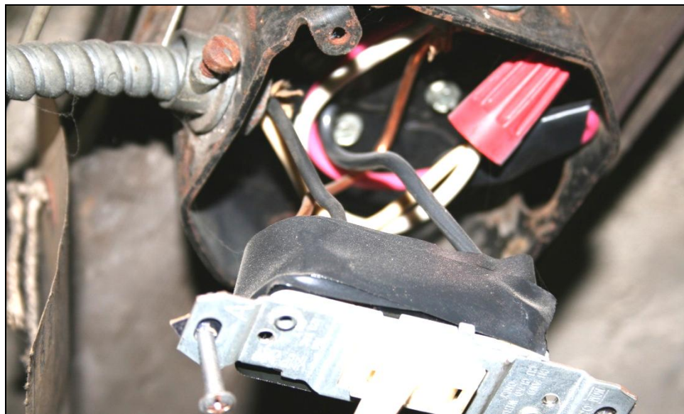
Inspection V53442: The switch is not installed in the proper switch box, exposing electrical wiring. This violation was not identified during the Authority's January 7, 2008, inspection.
