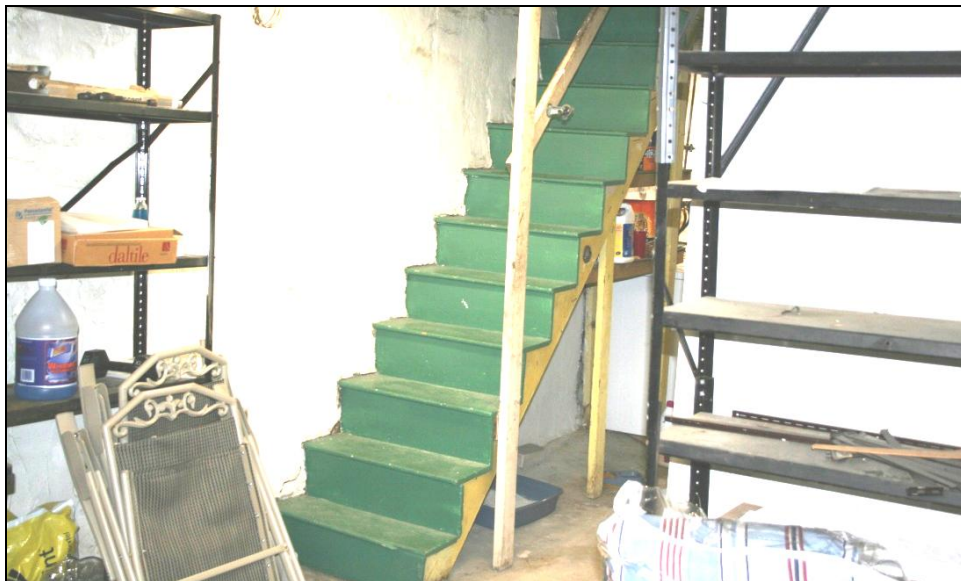
Inspection V07006: The handrail is not running the full length of the basement stairs. This violation was not identified during the Authority's December 12, 2007, inspection.
