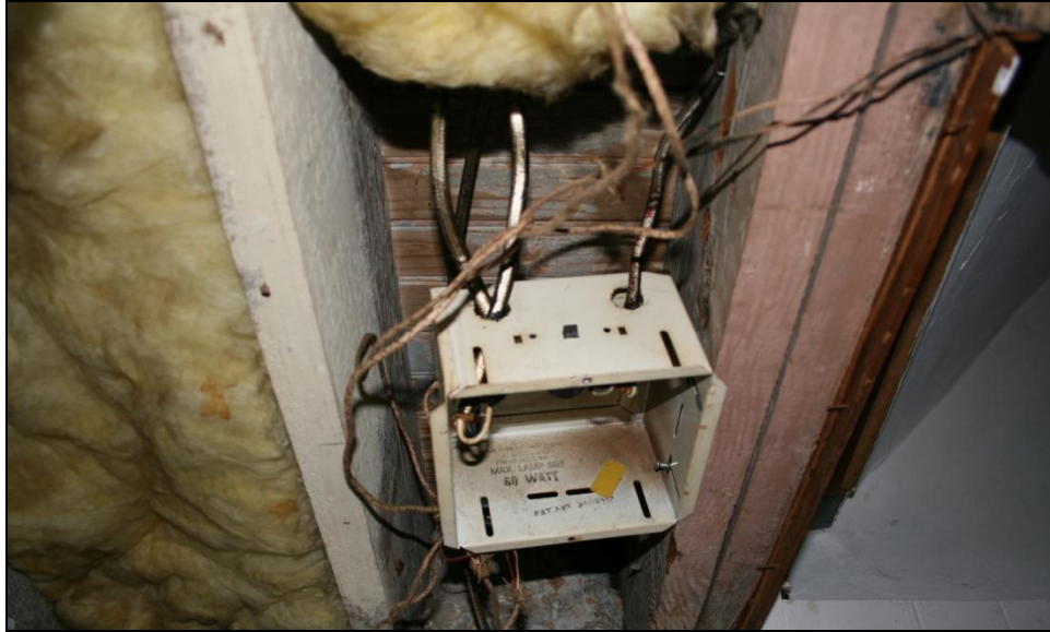
Inspection V54218: The recessed light fixture at the base of stairs is not secure and wires are exposed. This violation was not identified during the Authority's November 21, 2007, inspection.
