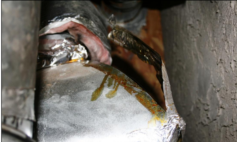
Inspection V73332: Improper and poor ventilation of the heating and air conditioning unit allows harmful gases to seep back into the basement. This violation was not identified during the Authority's January 28, 2008, inspection.
