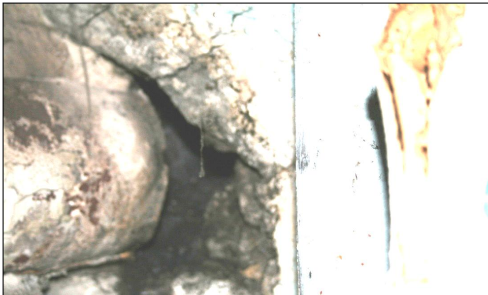
Inspection V45074: The furnace flue is disconnected from the wall, allowing harmful gases back into the basement. This violation was not identified during the Authority's November 28, 2007, inspection.
