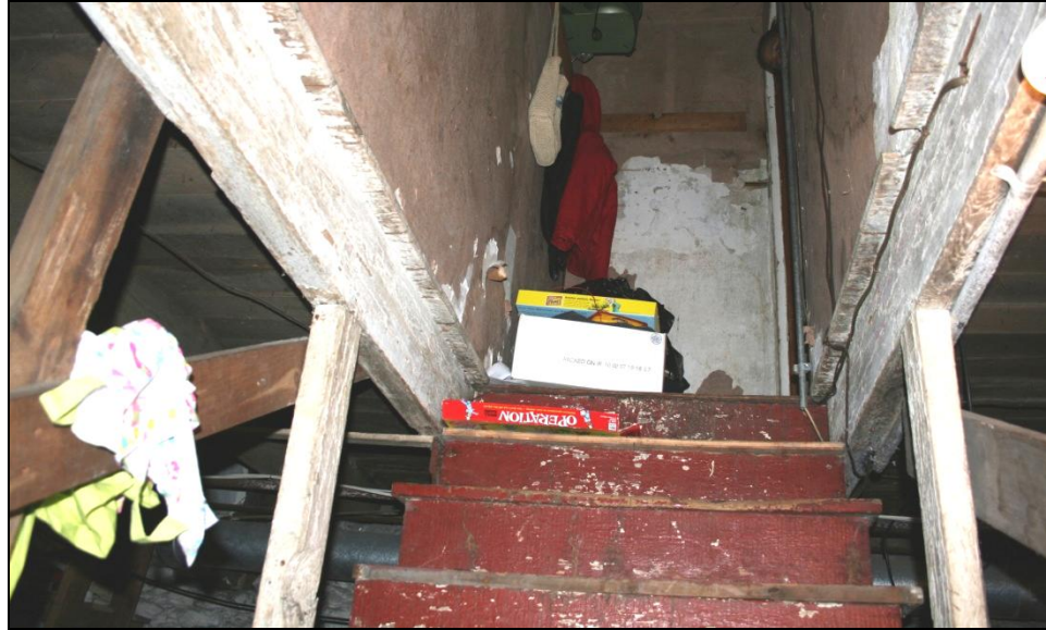
Inspection V73712: The handrail is not running the full length of the basement stairs. This violation was not identified during the Authority's December 10, 2007, inspection.
