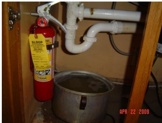
Leaking kitchen sink with a pot to contain the water
