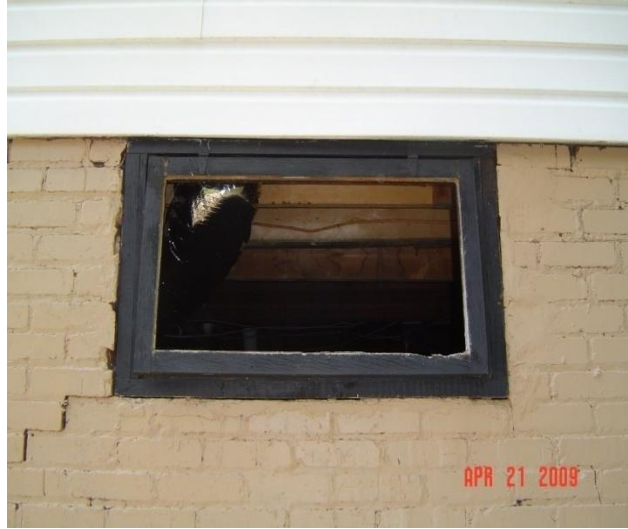
Cracked foundation and missing window pane in crawlspace
