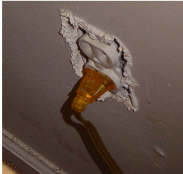
Missing outlet cover
