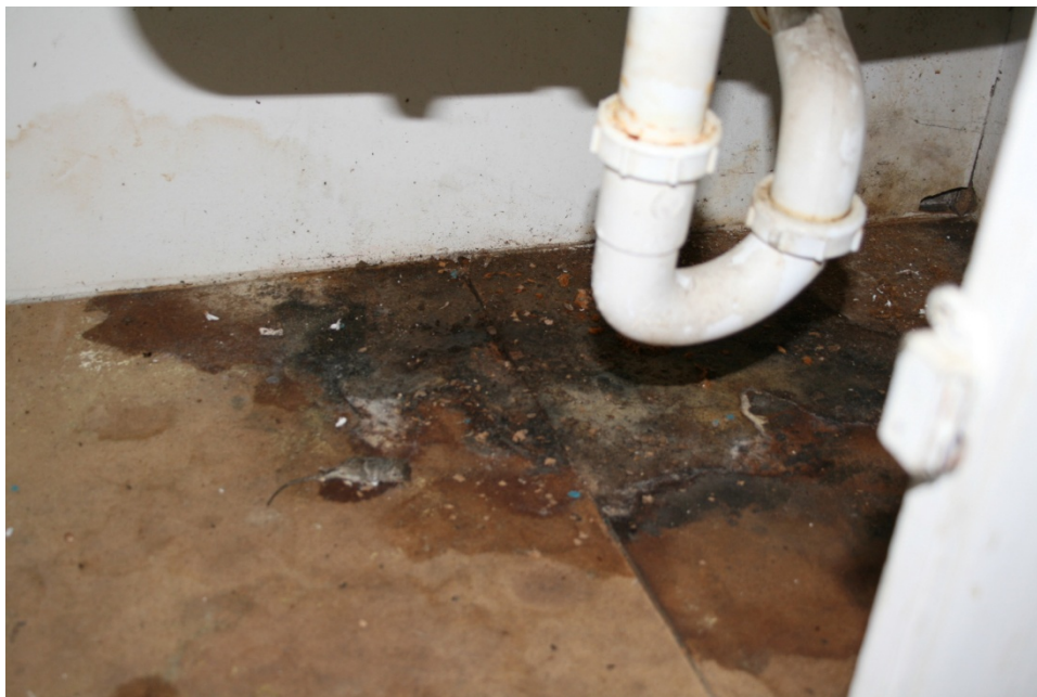
Infestation violation in unit 1523: There is a dead mouse under the kitchen sink.
