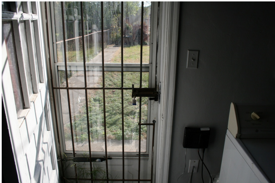
Door violation in unit 1905: A fire hazard is created by the burglar bars on the rear door. The tenant did not have the key to the padlock.
