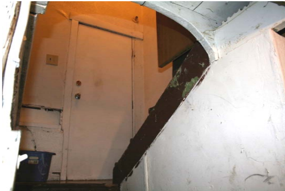
Stairs/porch violation in unit 5: The left side of the basement stairs needs railing to prevent tenants from falling down the second flight of stairs.
