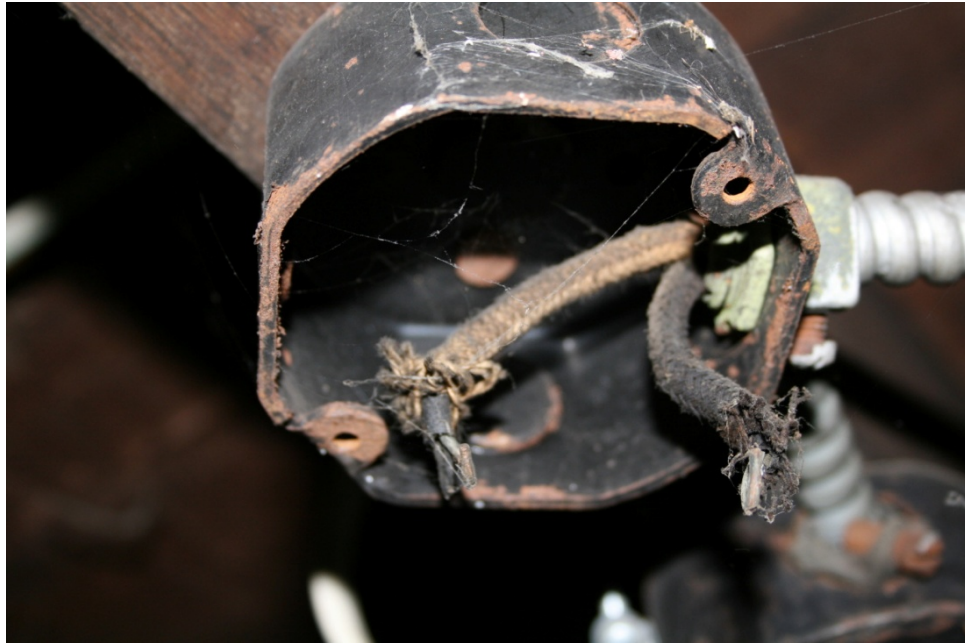
Electrical violation in unit 1302: The junction box contains exposed hot wires.
