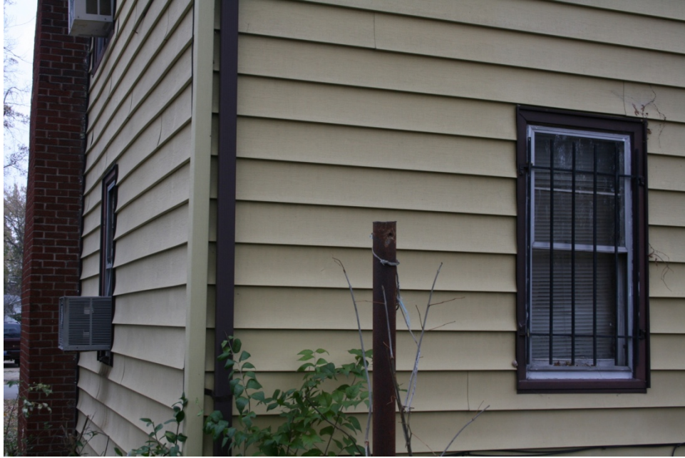
Window violation in unit 1383: A trapping hazard in event of fire was created by the burglar bars on the rear bedroom window and the air conditioning unit on the other window.
