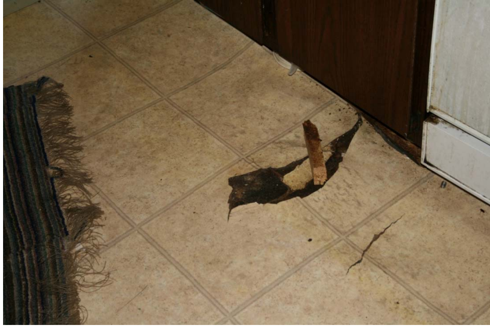
Floor condition violation in unit 1038: The vinyl kitchen flooring is torn, and the subfloor is rotten and spongy.
