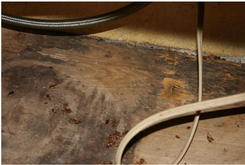
Units had evidence of roach infestations.
