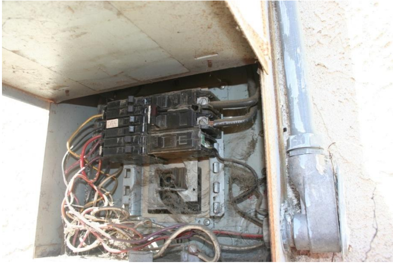
Main service panels were missing the interior safety panels, exposing electrical wiring.
