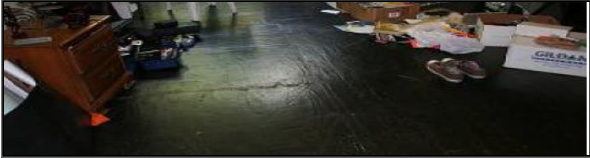
None of the 30 units had carpets installed as indicated in the scope of work.
