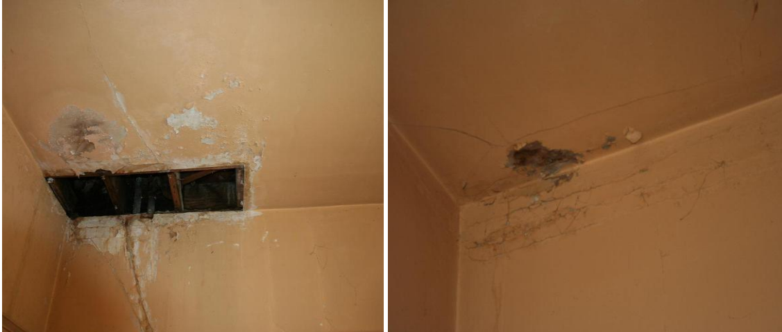
Project #2106: Room not rehabilitated despite ceiling and wall damage
