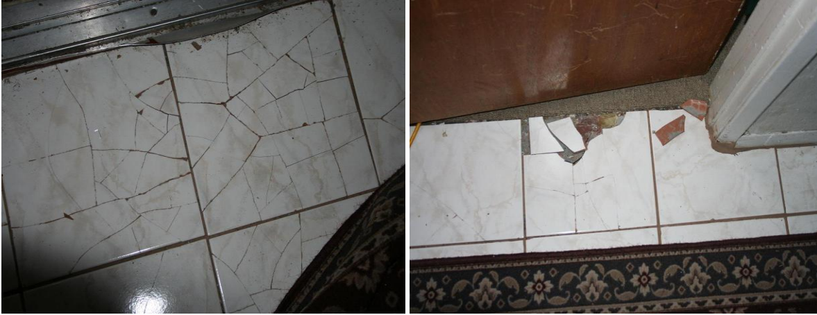
Project #1946: Tile flooring cracks in kitchen and hallway due to improper installation
