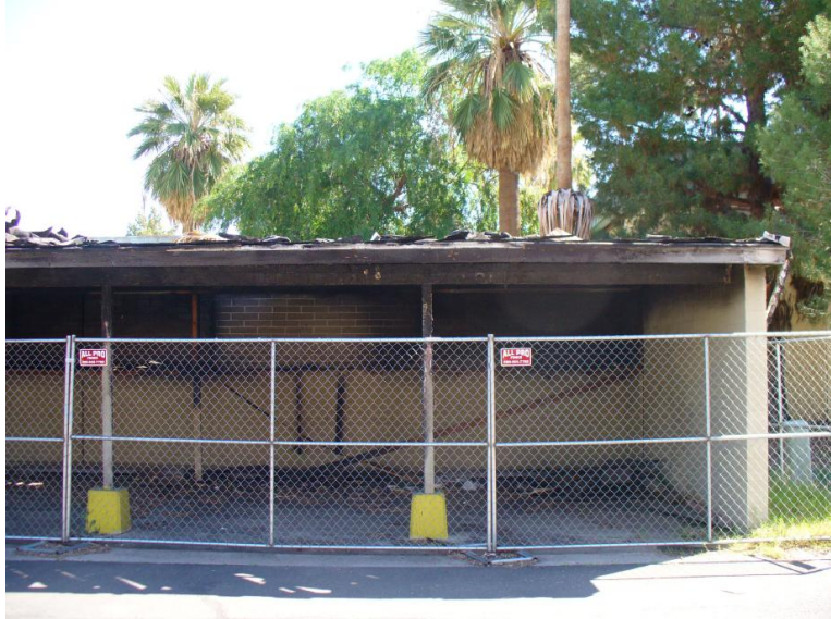
This carport was damaged by a fire that had occurred more than one year earlier.
