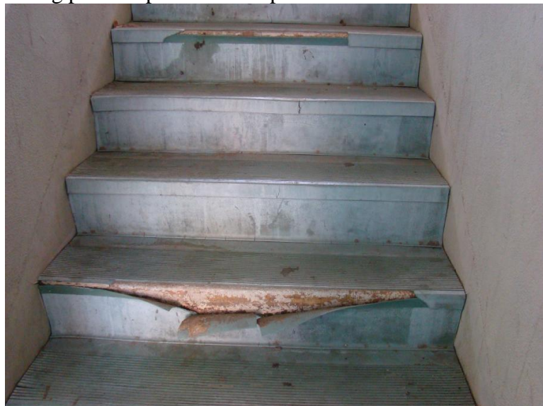
The building stairs had covering that was peeling.
