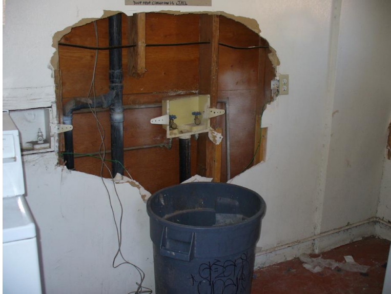
Multiple laundry facilities had holes in the walls.
