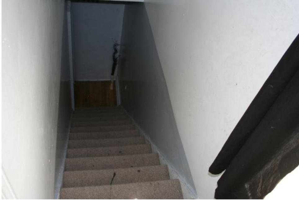
The interior hall staircase from the first to second floor had no handrail.
