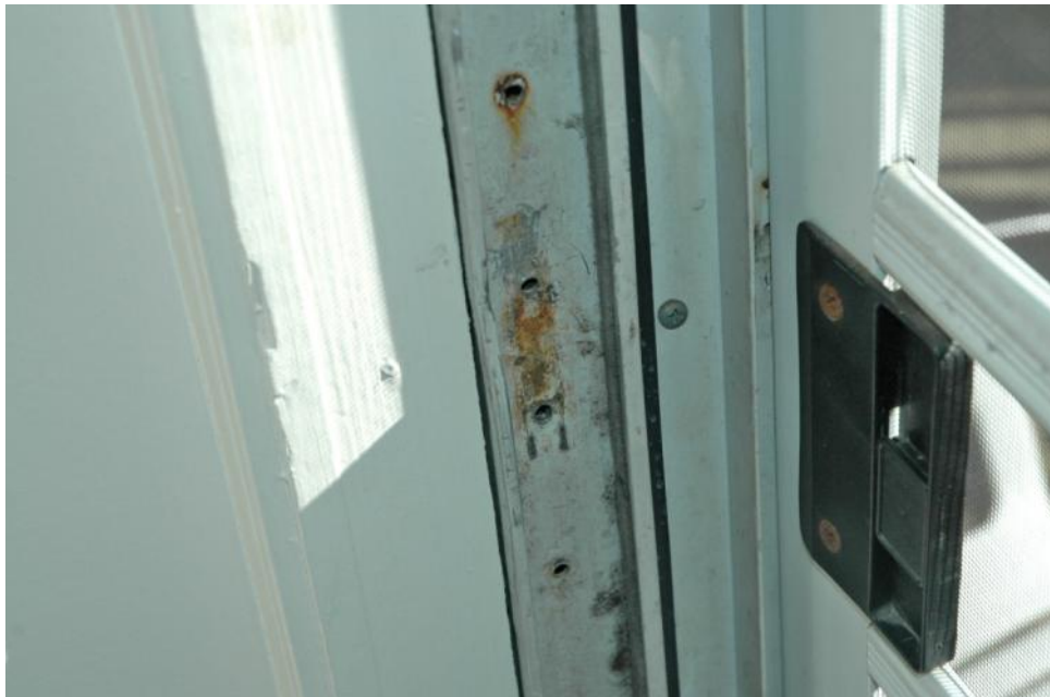
The missing lock hook from the patio doorframe did not allow the door to be properly secured.
