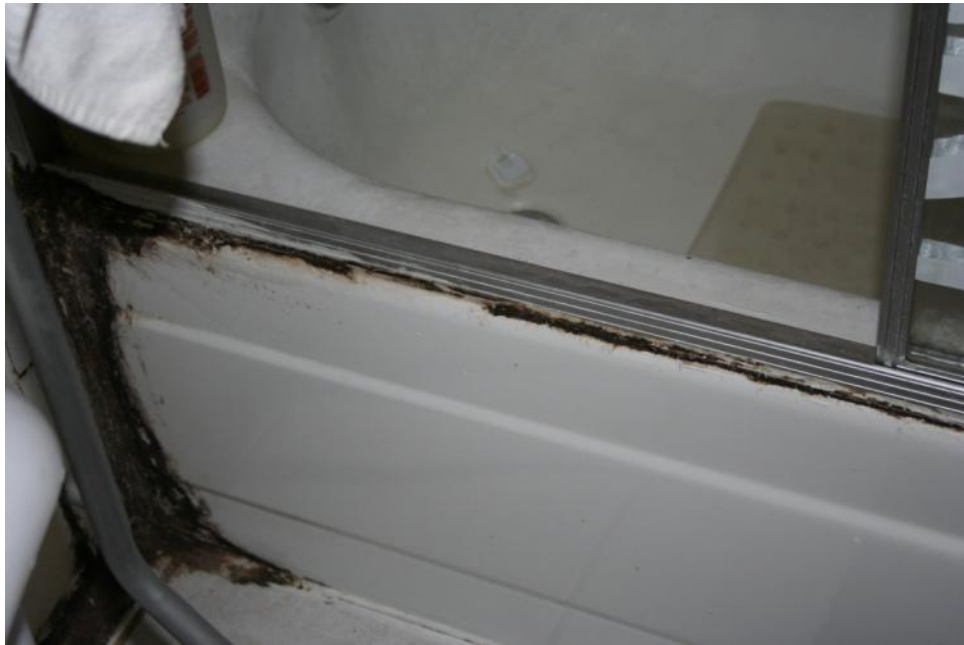
The tub, tile, and walls had excessive mildew buildup.
