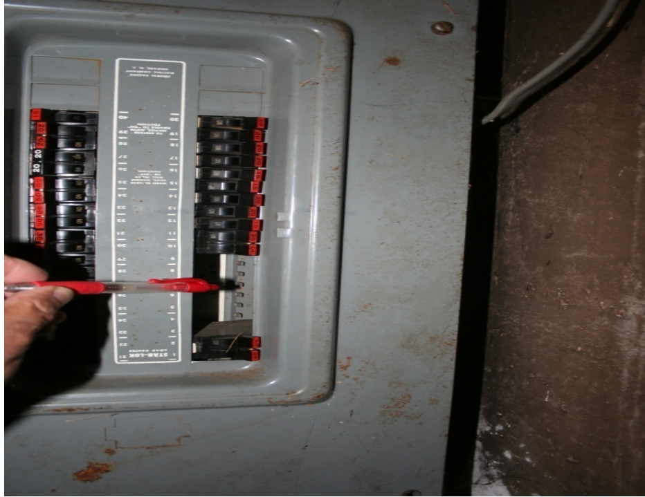
The electrical panel on the basement wall was missing seven breakers, exposing electrical contacts.
