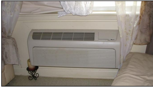
New energy-efficient heating/cooling unit installed in 2008
