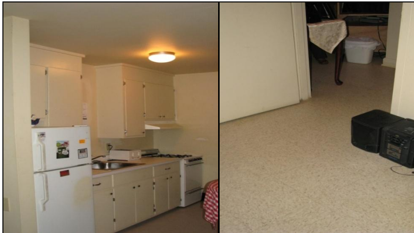
Kitchen cabinets installed in 2007
