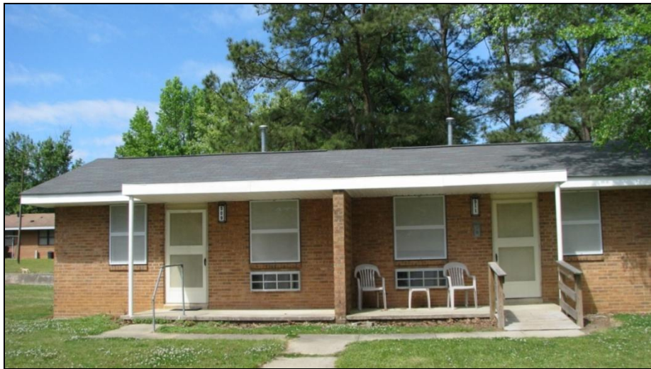
Forrest Road units – Note the new roofs, heating/cooling units, and windows installed in 2007 and 2008.
